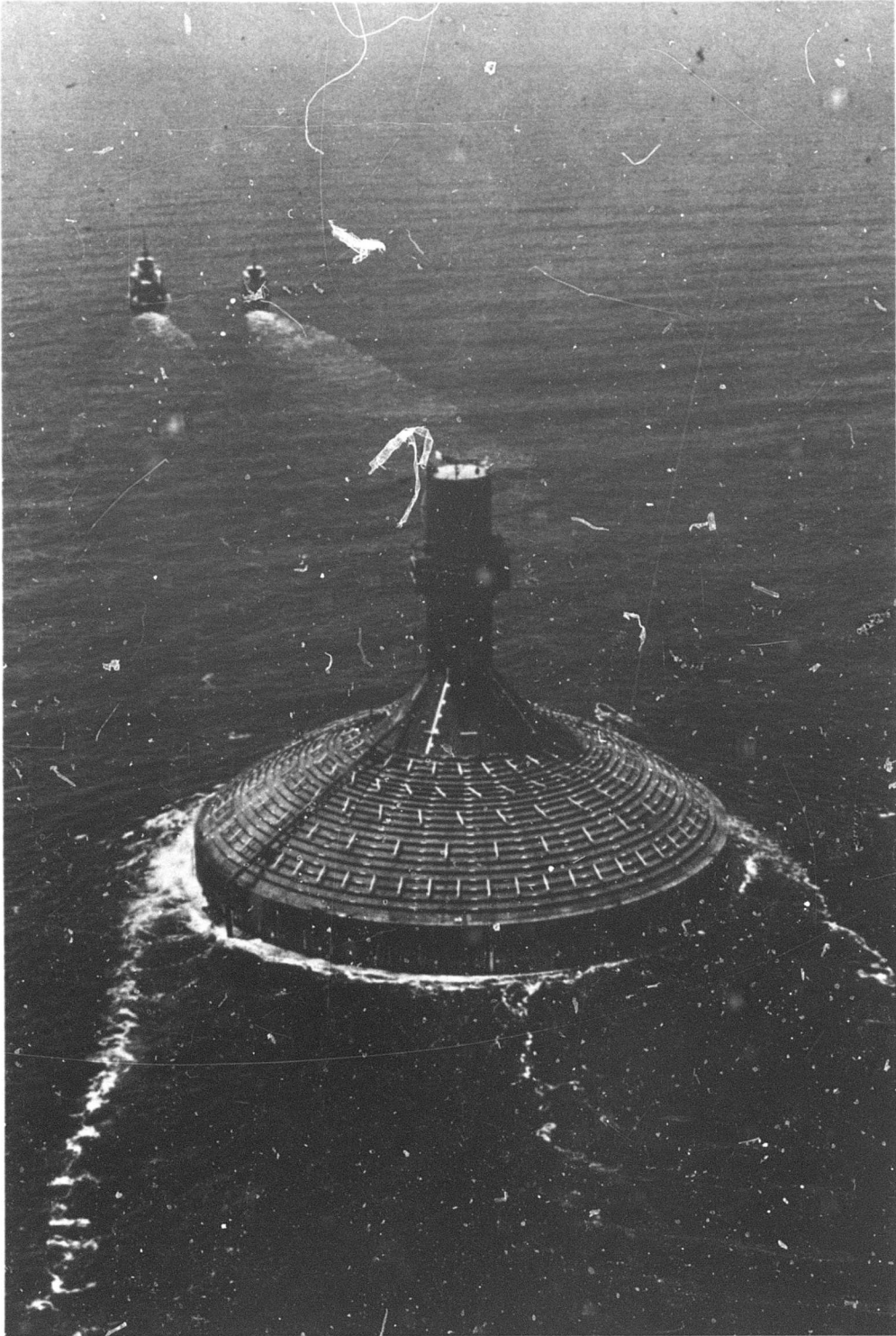
Figure 37. Khazzan Dubai I being towed to site. (From Chicago Bridge and Iron, 1969. Photo courtesy of Chicago Bridge and Iron Company.)
