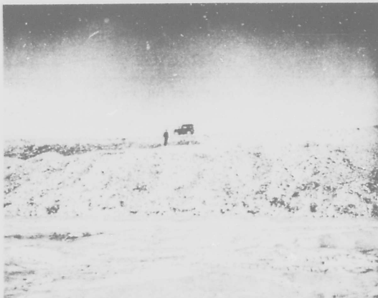
Figure 13. South side of Ramp Road, Station 4+00, 27 August 1959.
