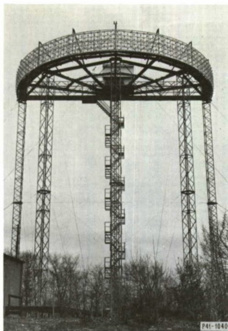
Fig. 1(a). Electronically scanned antenna for use with advanced MTI radar.
