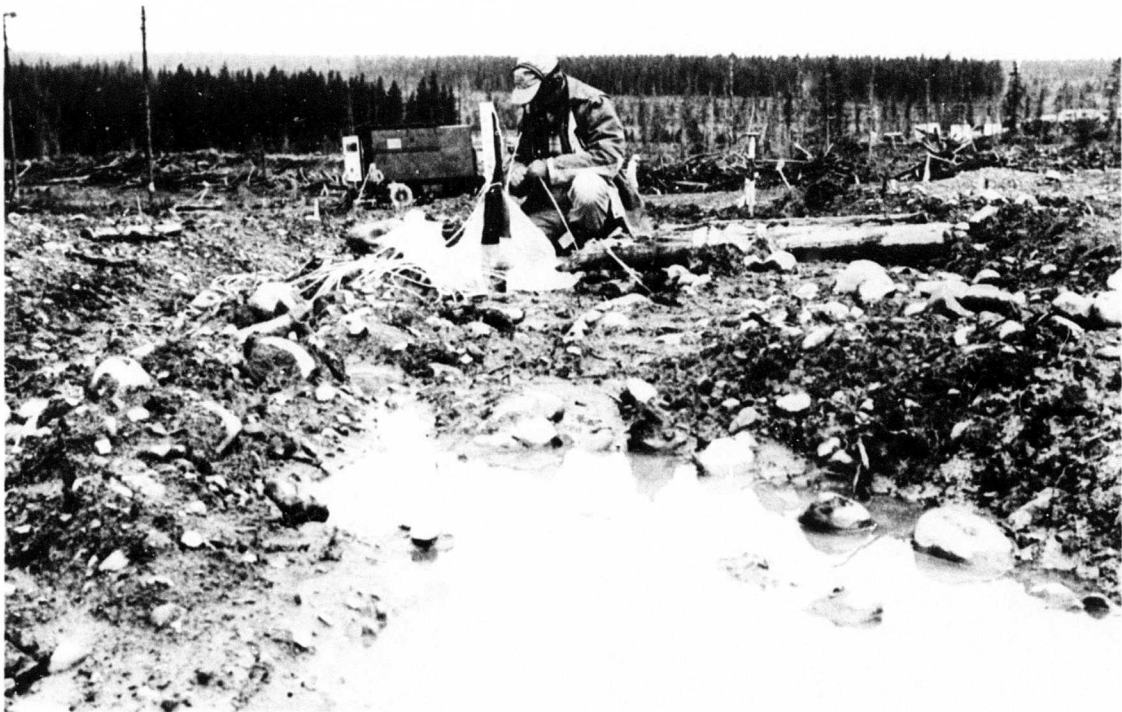
Figure 2.8 Photograph of cleared sector main blast line from GZ, preshot, Event 4.
