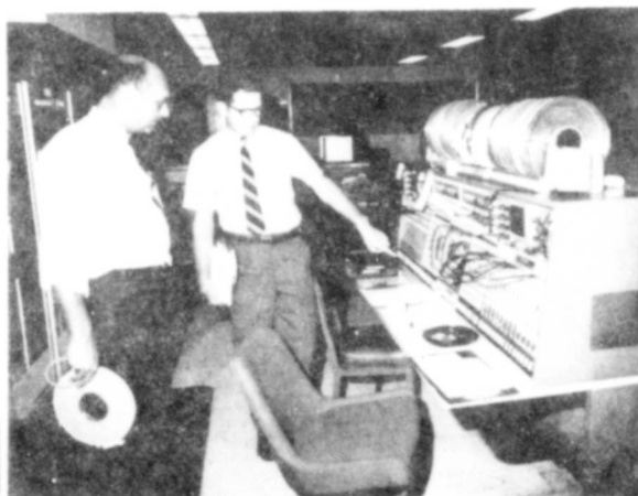
Figure 2. A view of the DDHS mode selection and signal-monitoring console.
