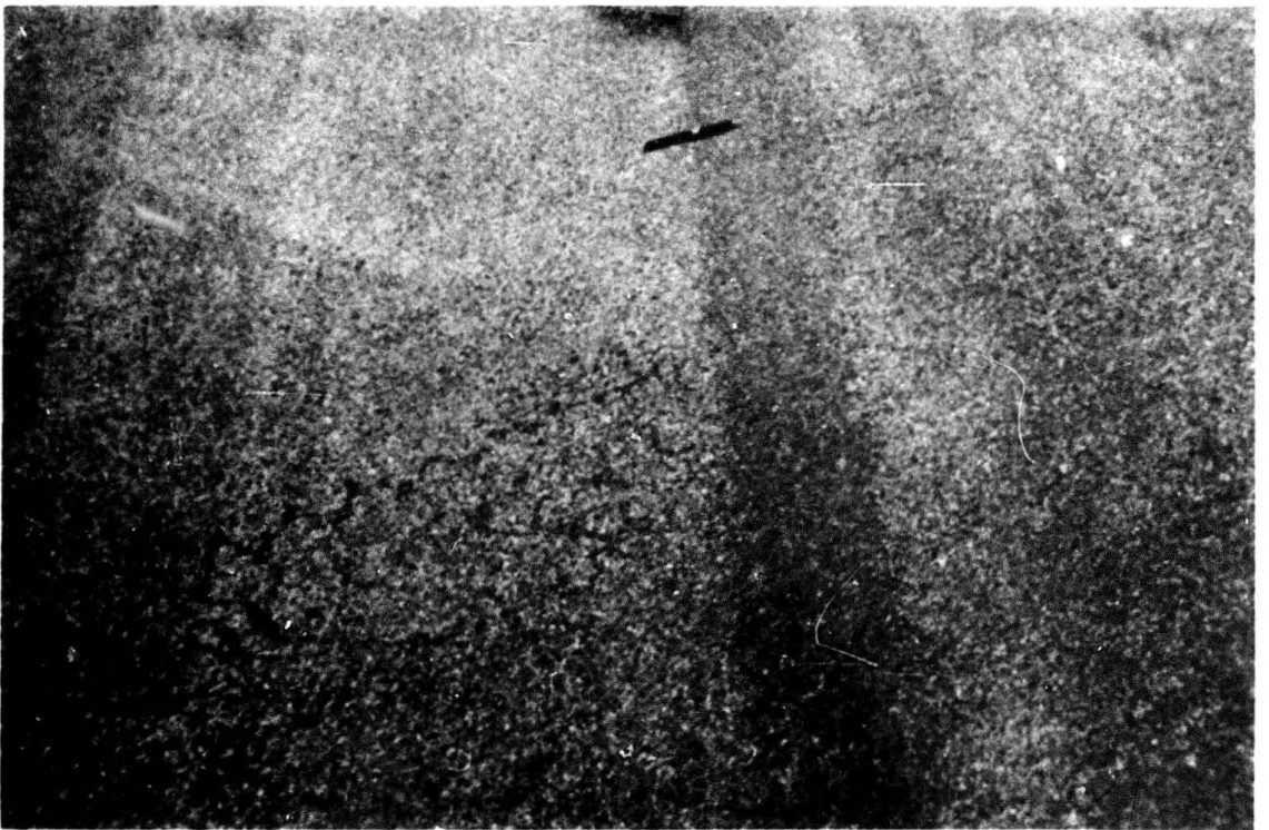
Photograph 6. Condition of pavement surface on east connecting taxiway near intersection with primary runway
