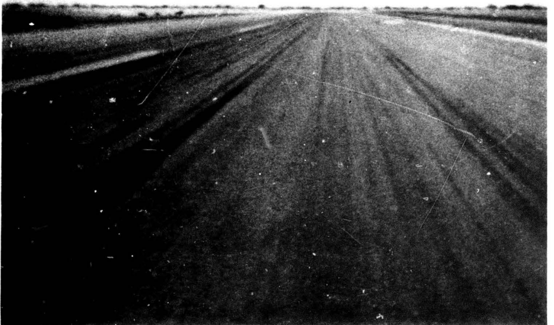
Photograph 2. View to northwest near center of primary runway. Note the birdbath near right edge of runway
