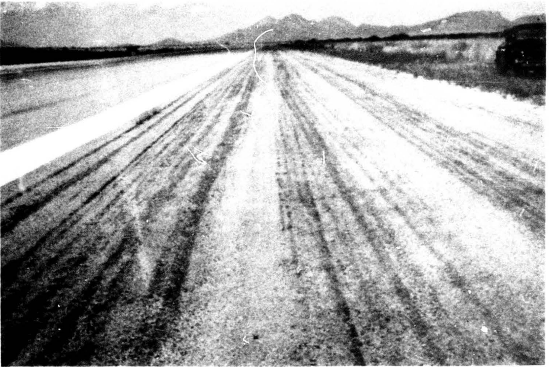
Photograph 3. Sand seal on surface of shoulder area along primary runway
