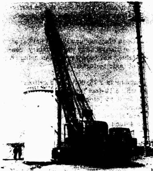
Fig. 15 - Facility Chamber Prior to Underground Installation
