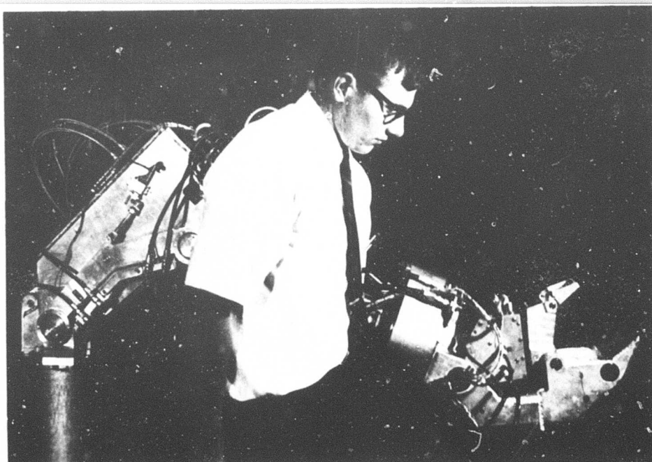
Figure 6. Part of General Electric's exoskeleton device.
