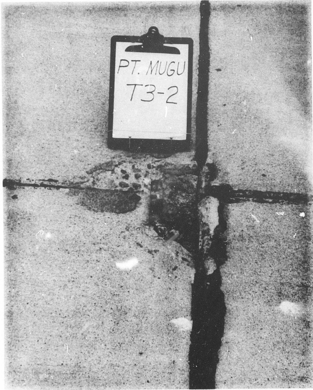
Figure 6. Failed corner spall repair, discrete area T3-2.
