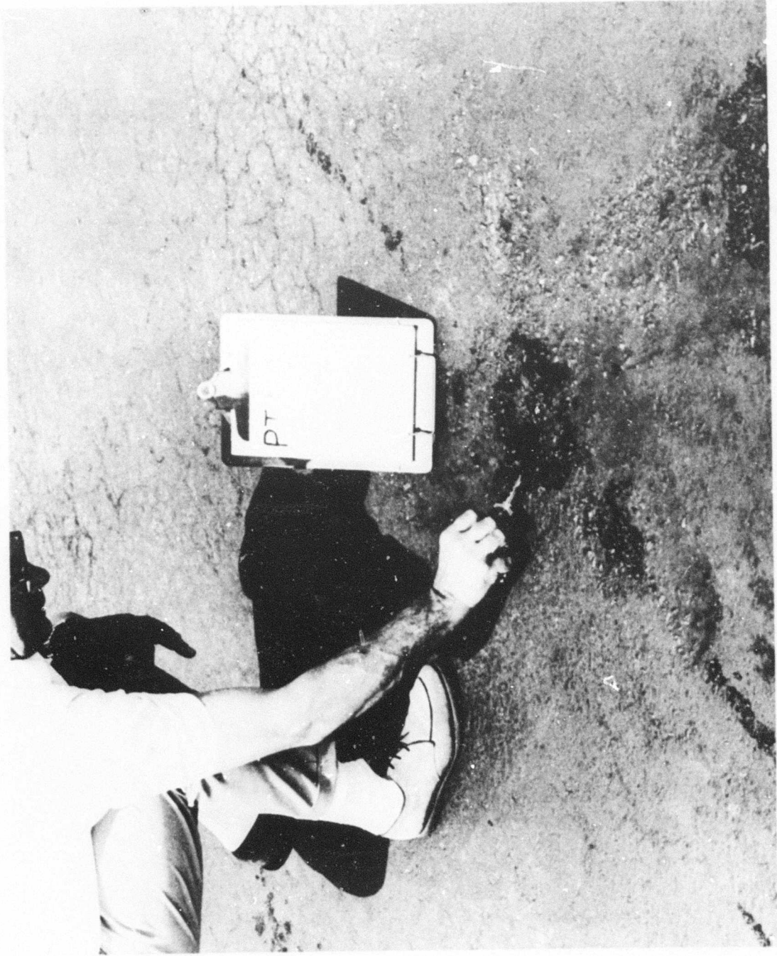
Figure 22. Surface softened by fuel or oil spillage, discrete area PA6-2.
