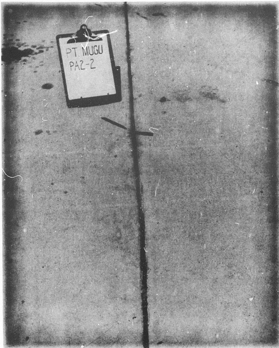
Figure 7. Missing joint seal, discrete area PA2-2.
