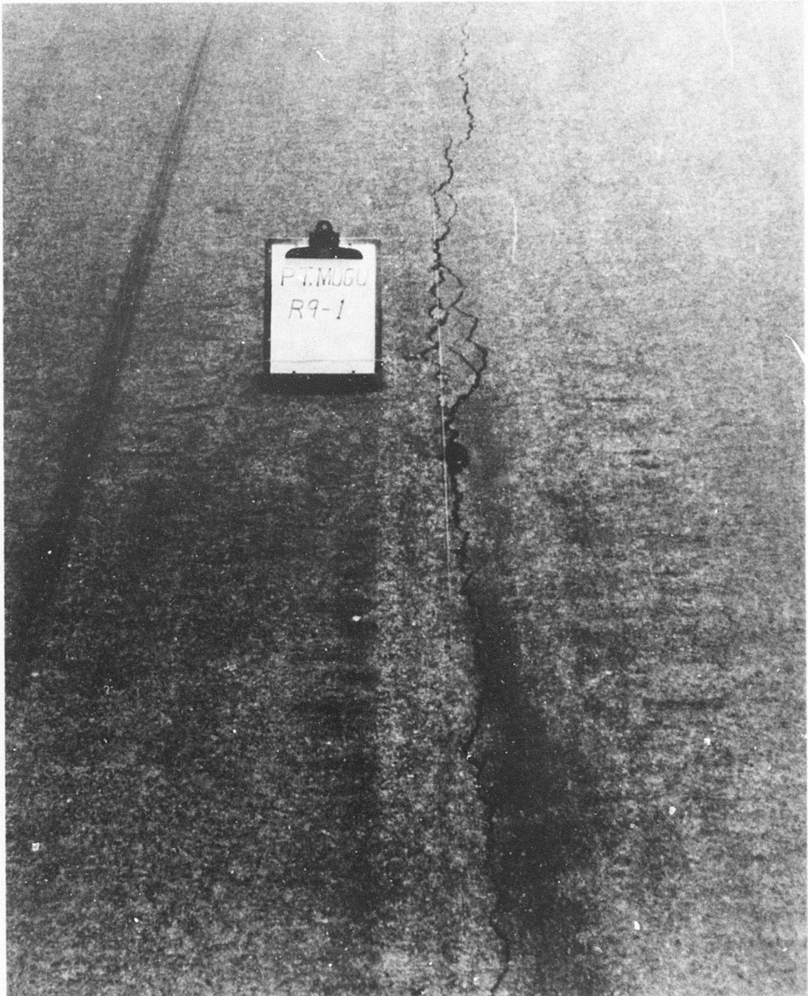
Figure 13. Unsealed longitudinal construction joint crack, discrete area R9-1.
