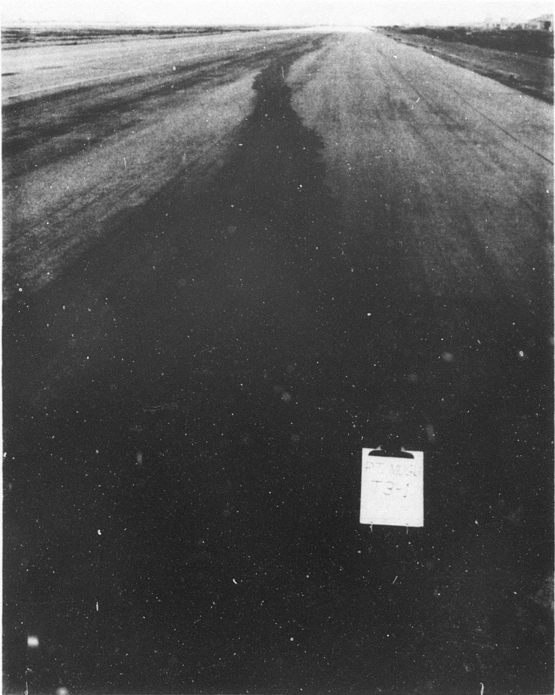
Figure 14. View of oil or fuel spillage, discrete area T3-1.
