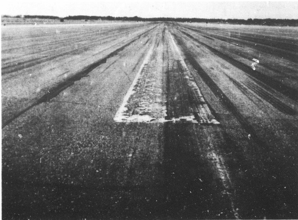
Figure 27. Deteriorated centerline striping at Oxnard Air Force Base, December 1969.
