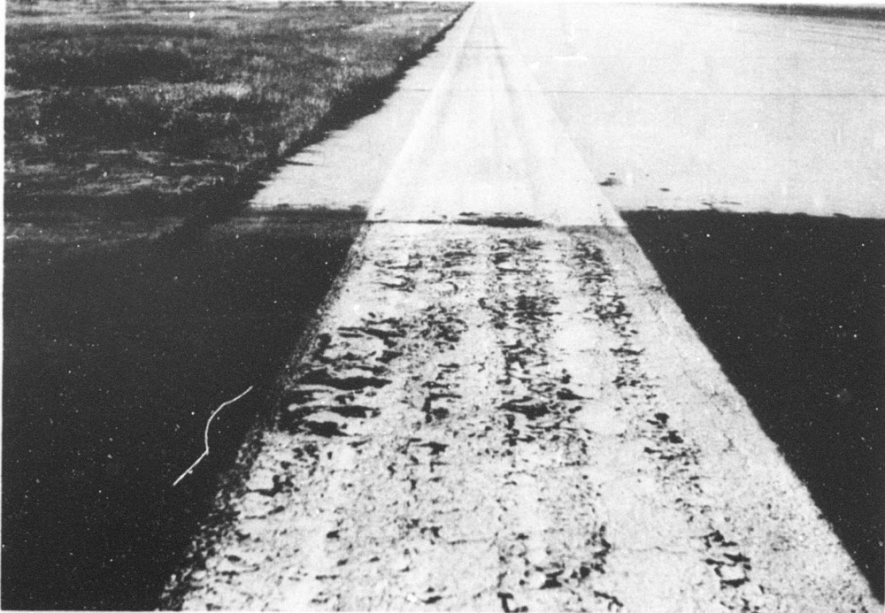
Figure 28. Deteriorated side line striping at Oxnard Air Force Base, December 1969. Note better condition of striping on portland cement concrete portion than on asphaltic portion.
