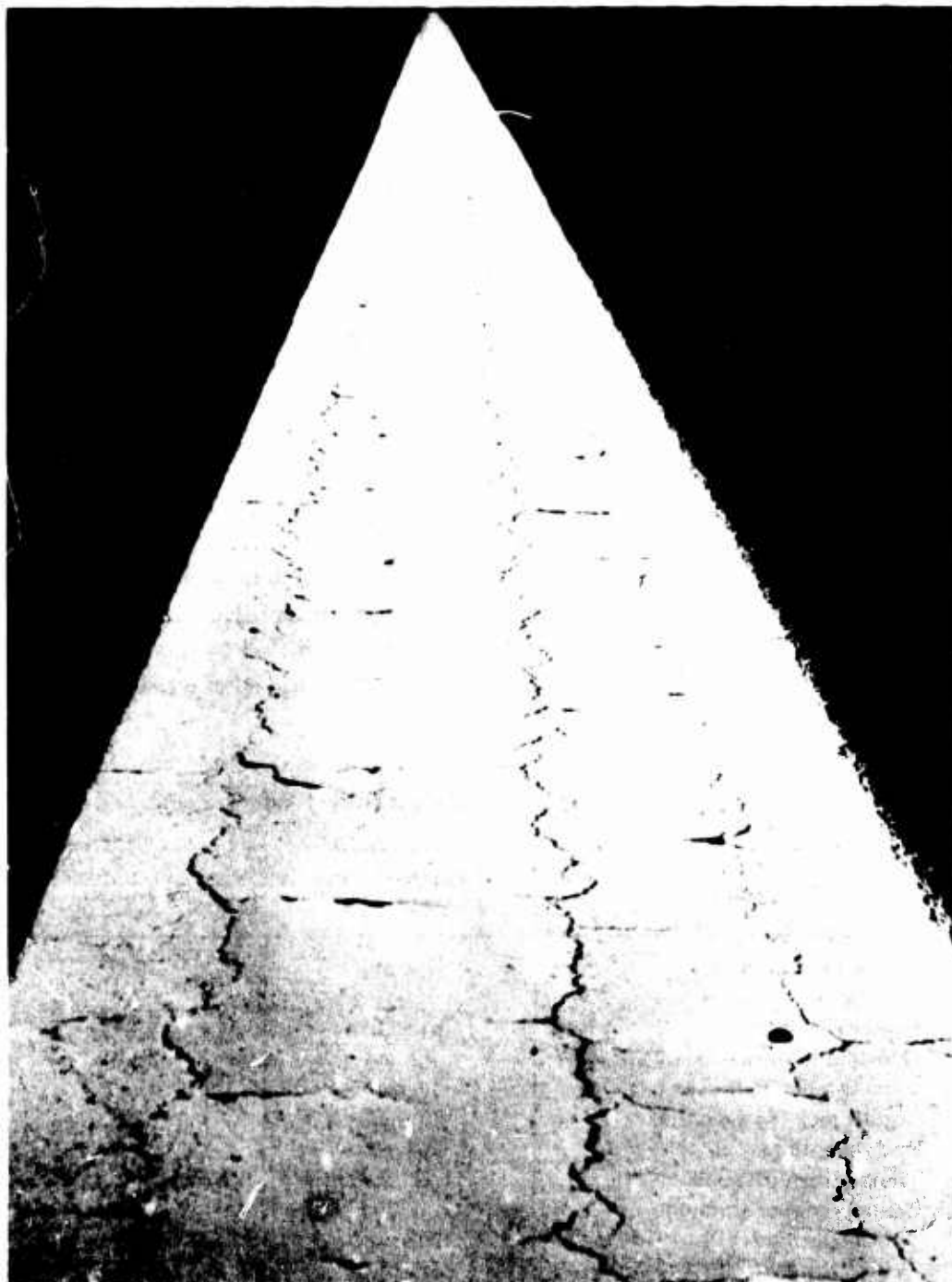
Figure 36. Deteriorated side line striping on Runway 17-35, MCAS, Yuma, in October 1968.
