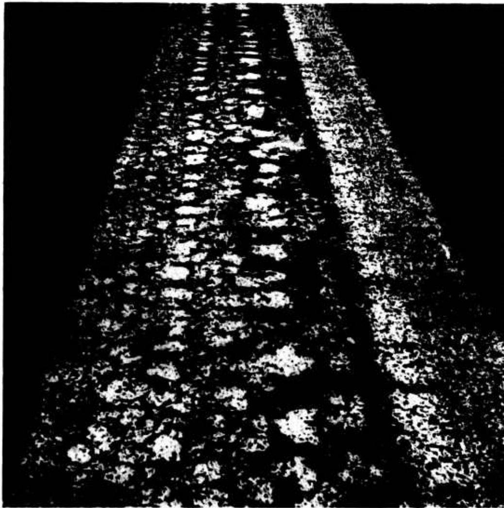
Figure 39. Deteriorated side line striping on asphaltic Runway 12-30 at San Nicolas Island.
