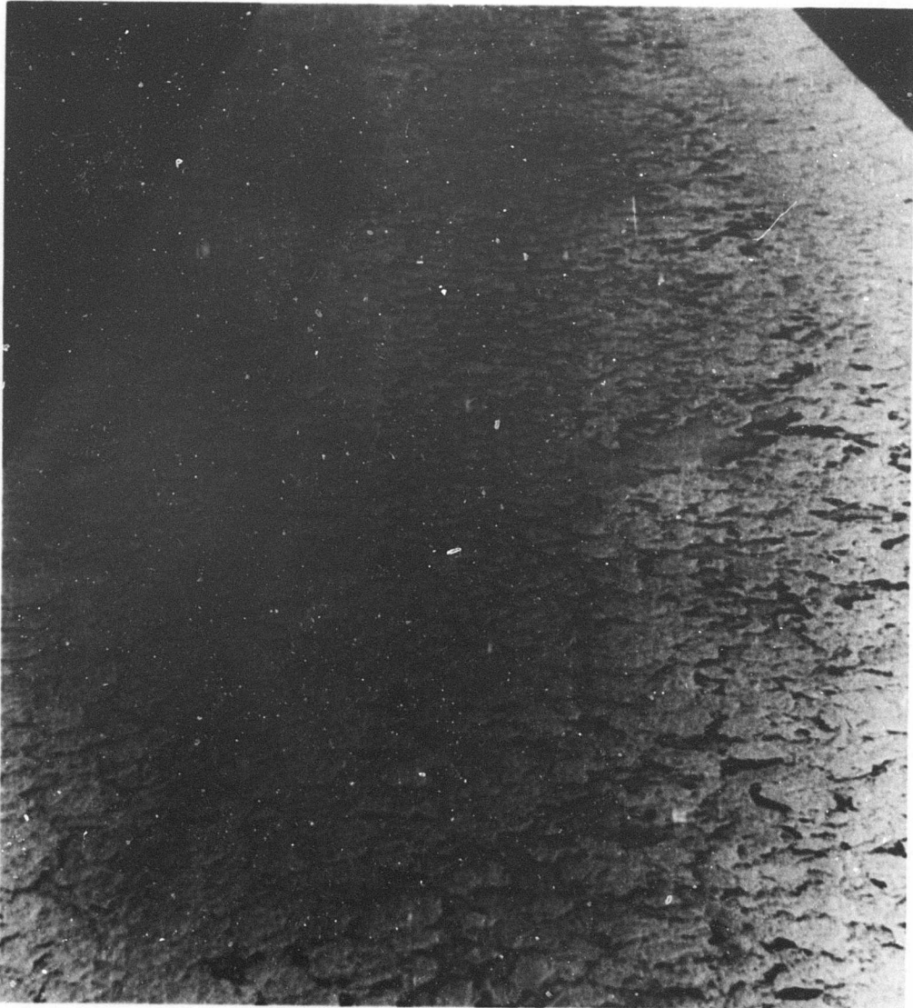
Figure 30. Airfield marking at NAS, Imperial Beach in August 1966, 10 months after striping.
