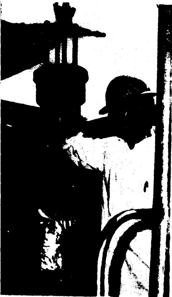
Figure 4d. Insertion of the end-closure assembly into the pressure vessel.
