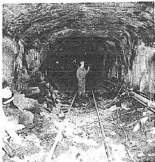
Figure 4. Post-test view in vicinity of Station 1.
