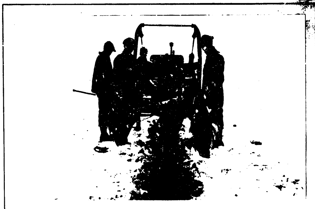
SLOT MADE IN FROZEN SOIL BY CABLE LAYING DEVICE
