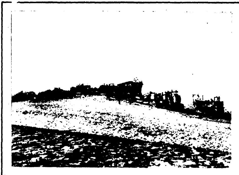
CABLE LAYING PLOW IN OPERATION
