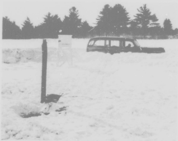
Thermocouple switch box installed. Steel cover removed to set rotary switch to obtain readings. Lead cable is to be connected to temperature indicator. Note plywood insulation cover.
