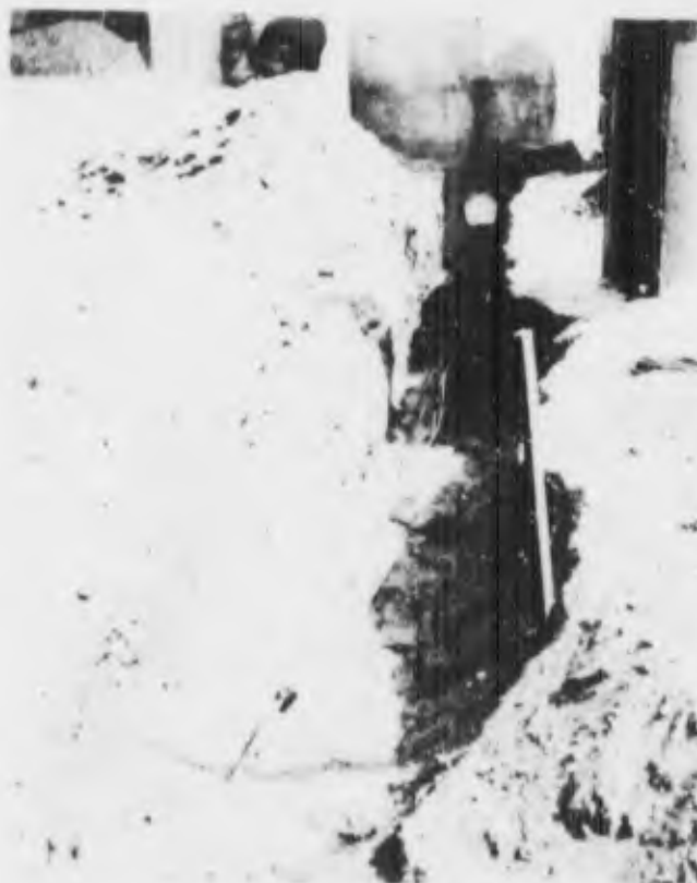
Figure 2. Thermocouple leads in trench from elements to instrument room
