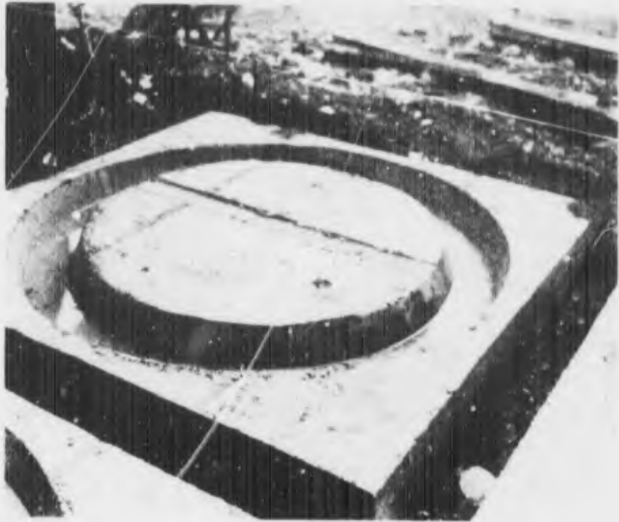
Figure 1. Detail of concrete foundation for Element A
