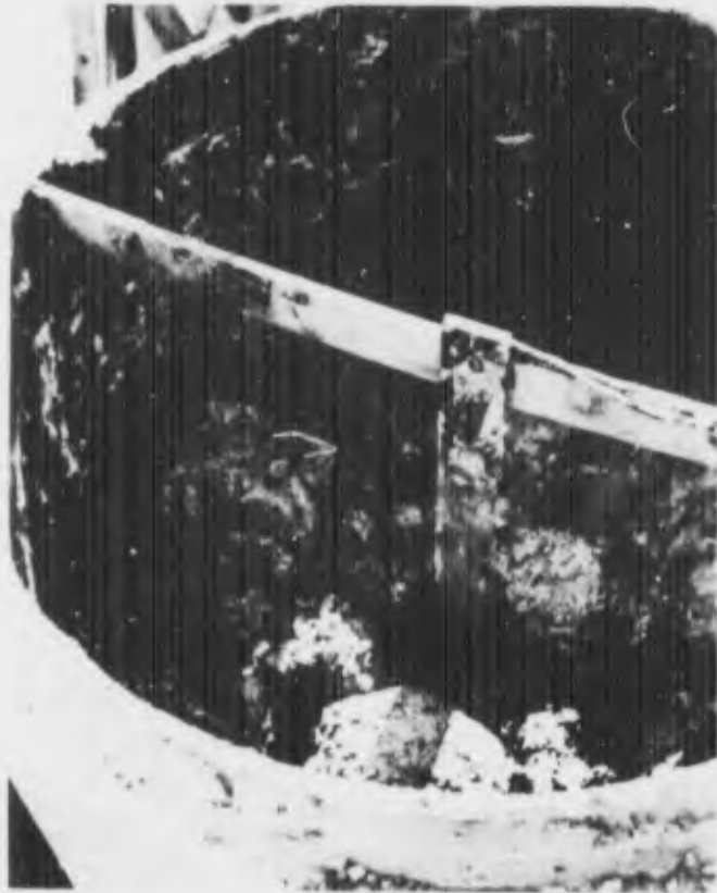
Figure 1. Subgrade material in element m_1 , placed at density of 90 PCF and at water content of 28 per cent
