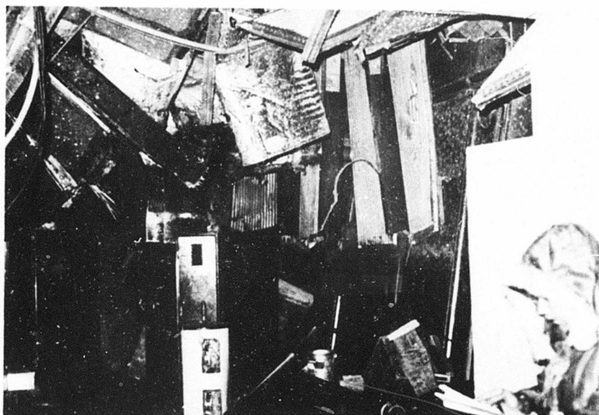
Figure 19. Deterioration of reactor building (Trench 5).
