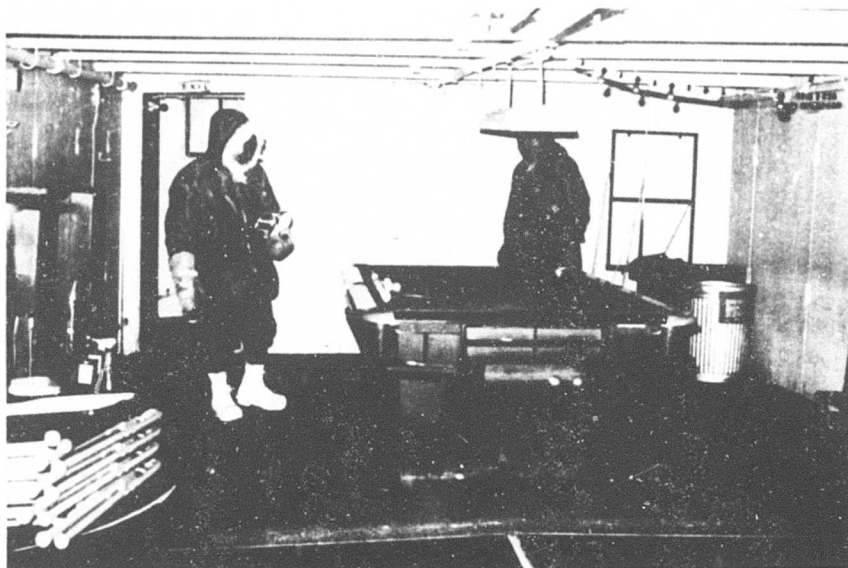
Figure 46. Floor buckling in EM club.
