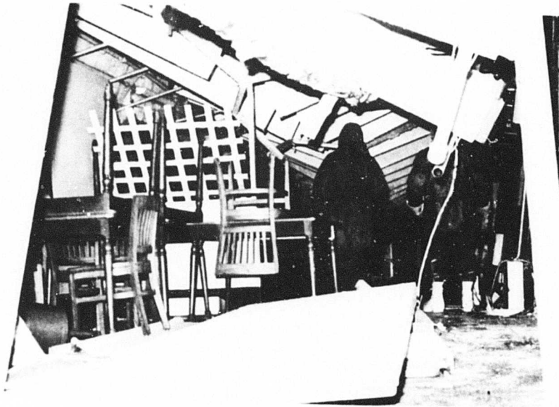
Figure 24. Ceiling joists pushed downward by snow encroachment upon mess hall roof.
