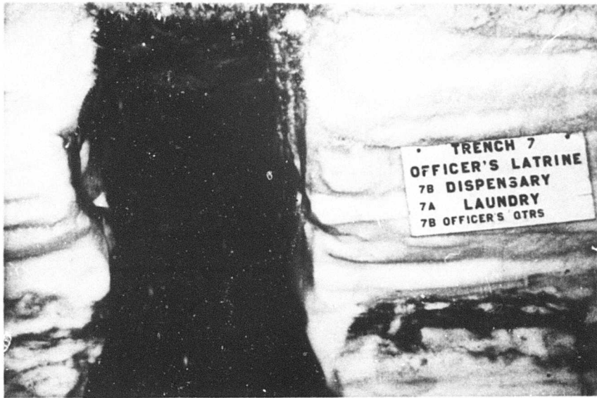
Figure 33. Entrance to Trench 7.
