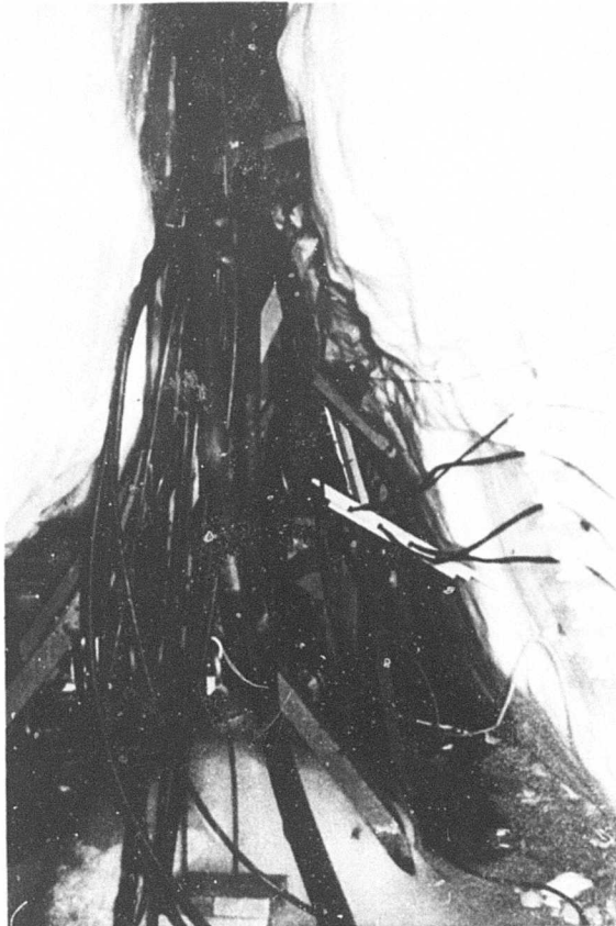
Figure 12. Snow deformation crushes the derrick over the glycol well.
