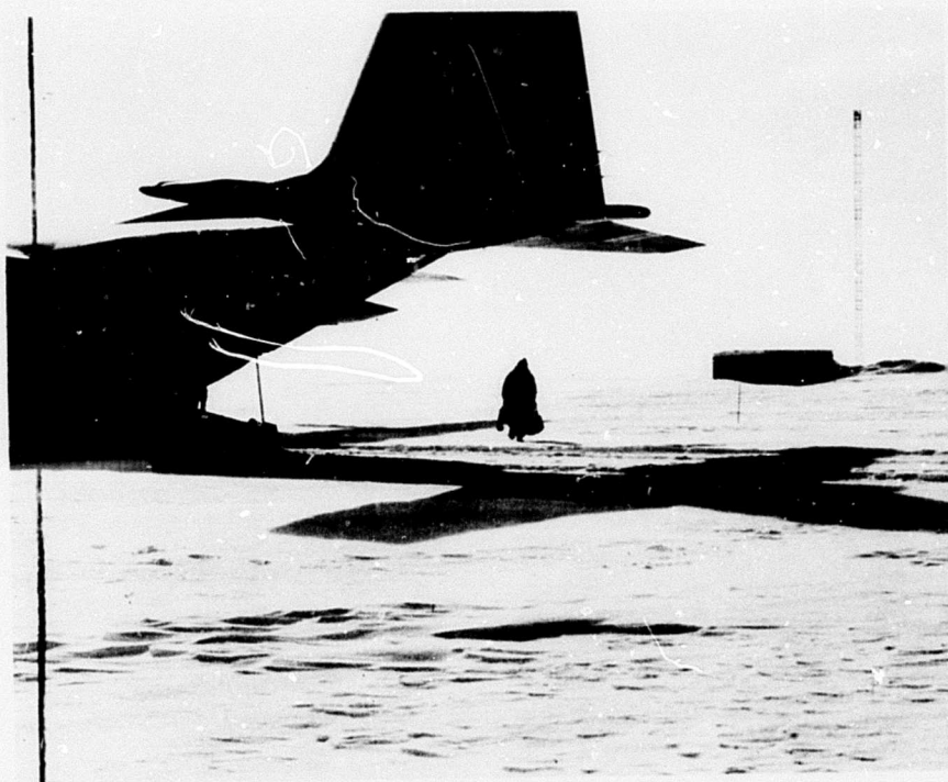
Figure 3. Arrival day. The structure protruding above the snow surface was built in 1964 on piles and was at that time 12 ft above the surrounding snow surface (see Fig. 4). This facility was occupied by the 1967 and 1969 field parties. In the background is the Sig. Met Tower.
