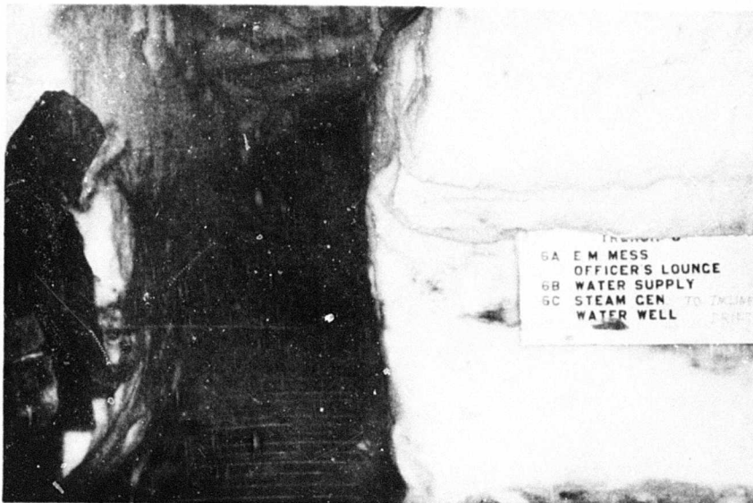
Figure 22. Entrance to Trench 6.
