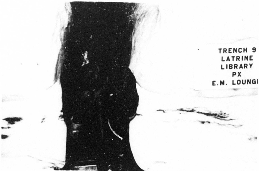
Figure 40. Entrance to Trench 9.
