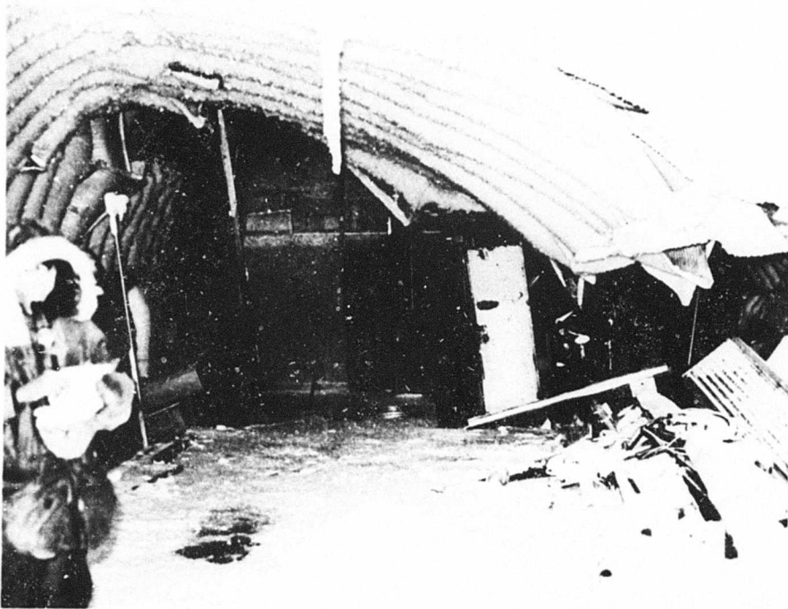
Figure 21. Metal arch buckling (Trench 5).
