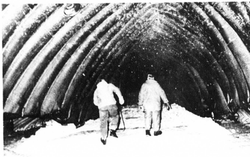
Figure 85. Steel arch deformation around maintenance shop.
