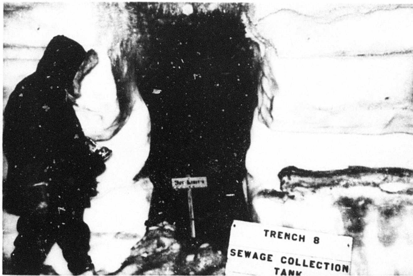
Figure 38. Entrance to Trench 8.
