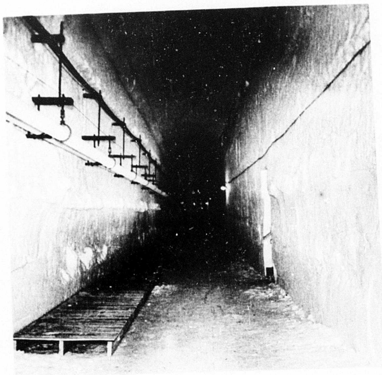
Figure 28a. Trench 6 passageway in 1960. (From Leighty, 1963).
