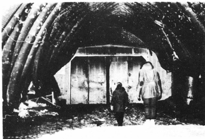
Figure 85. Steel arch deformation around maintenance shop.
