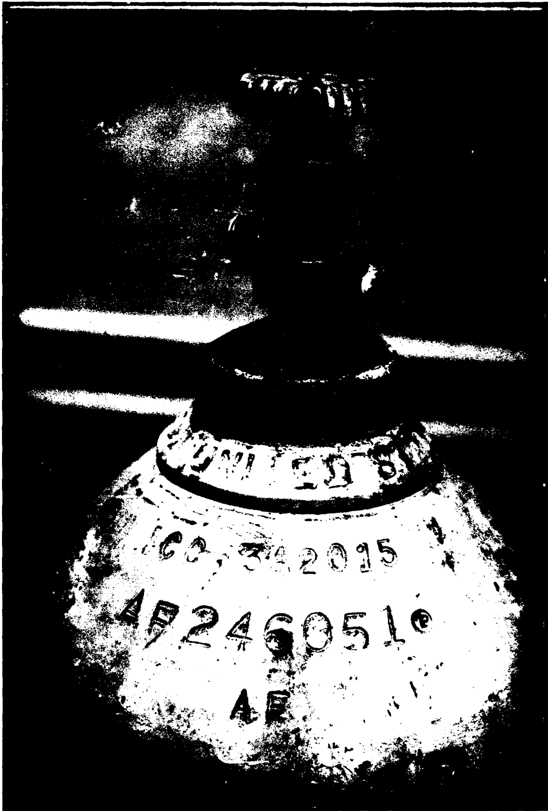
FIGURE 46 ICC MARK ON COMPRESSED-GAS BOTTLE
