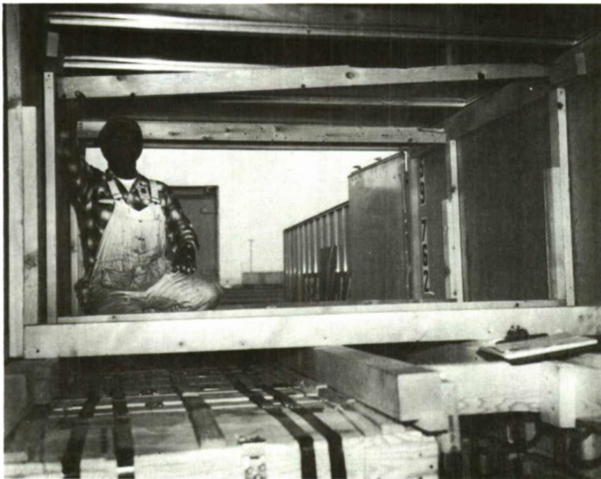
Figure 13. Container Number 59762, 2- by 4-Inch Spreader Overhead Needed To Be Replaced.
