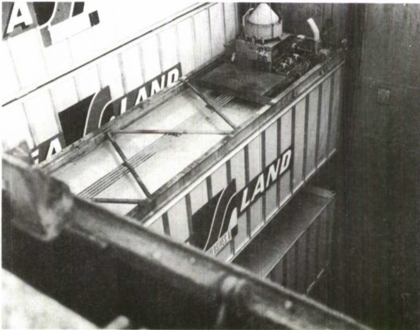
Figure 24. Container Being Lowered Into Final Position.
