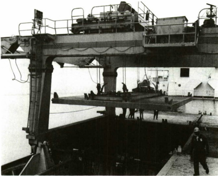
Figure 21. Removal of Hatch Cover by Gantry Crane.
