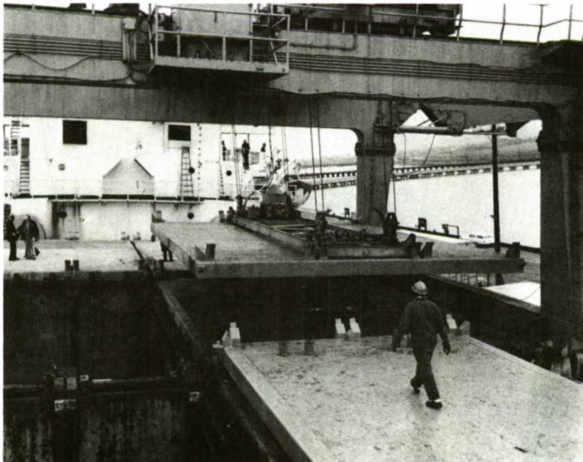
Figure 22. Hatch Cover Being Set Aside To Open New Hatch.
