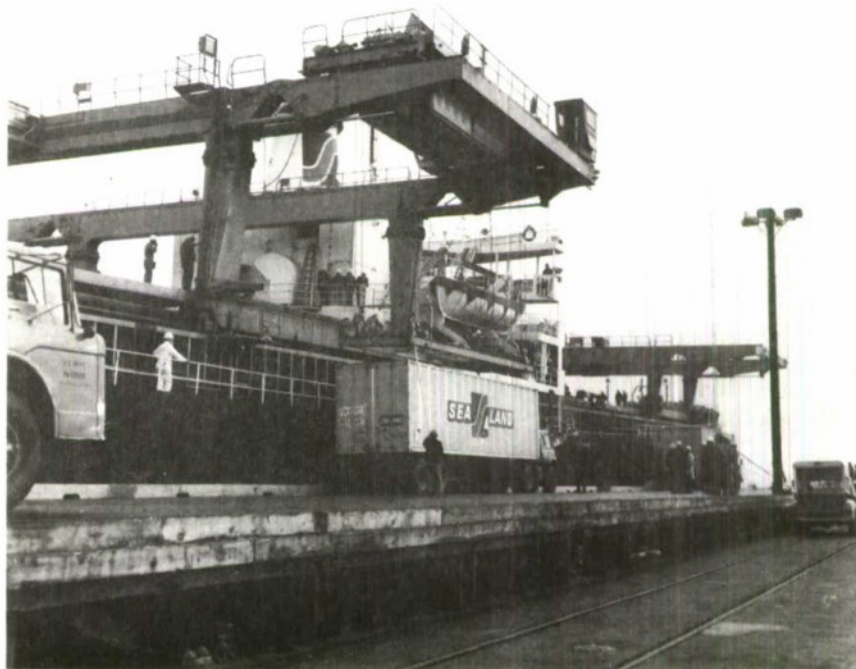
Figure 16. Aft Gantry Crane Spreader Frame Being Positioned, Using Boat Hooks for Lifting Container Aboard.
