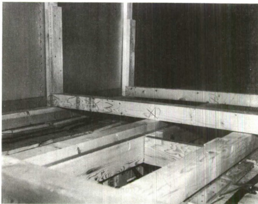
Figure 12. Container Number 59783, 4- by 4-Inch Bracing in Need of Nailing.
