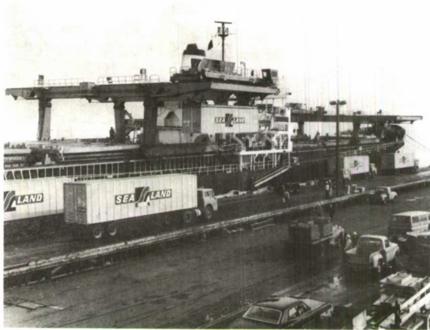
Figure 19. Container Lifted Full Height; Empty Trailer Bed Moving Out of Loading Position.
