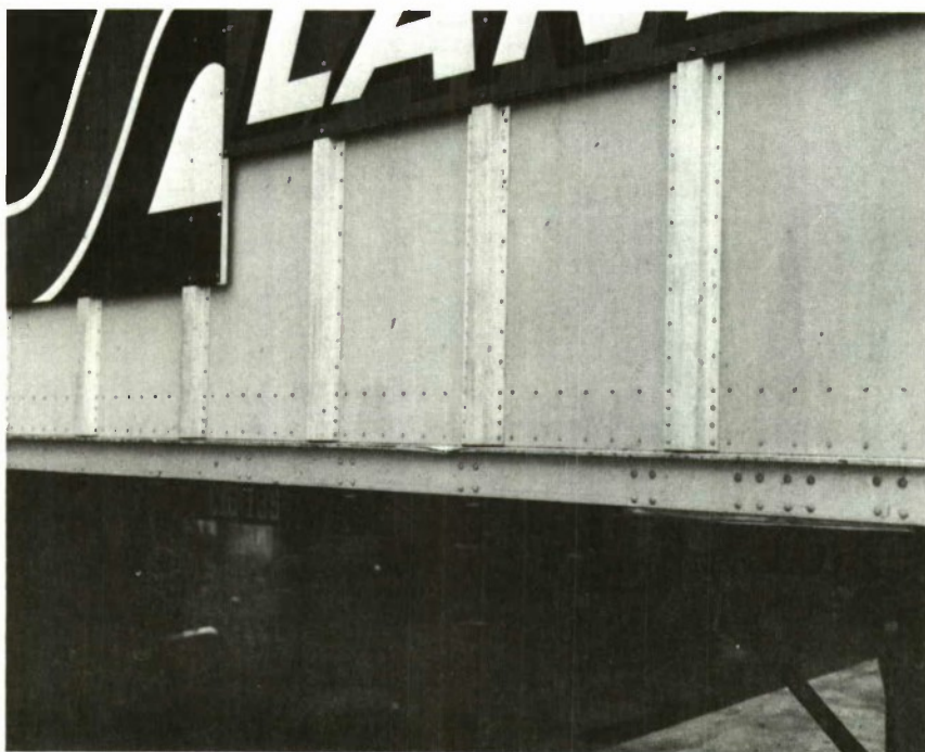
Figure 5. Minor Damage to Right Mid-Point of Frame.
