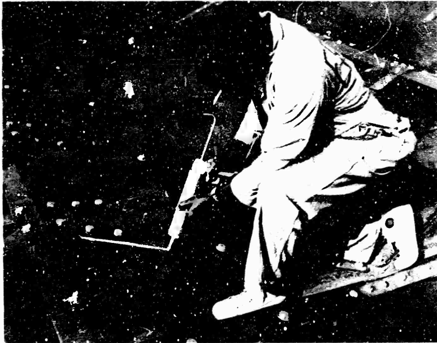
Fig. 44. Caulking application.
