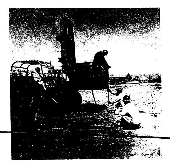
Figure 4. Installing rods with air hammer at NCEL test site.
