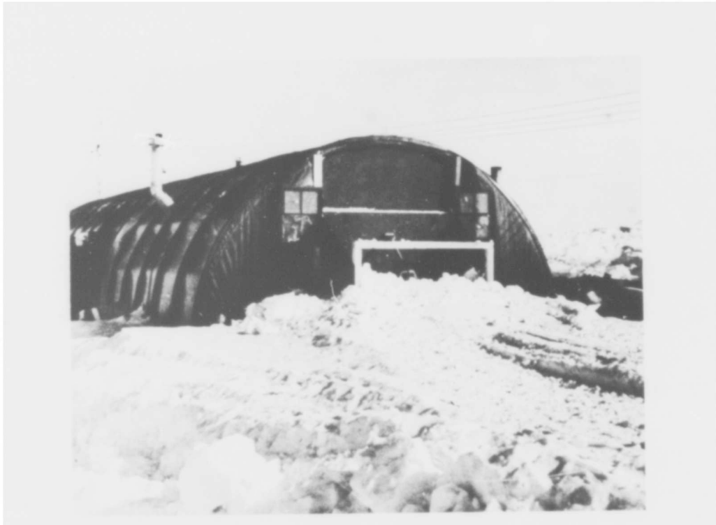
Figure 14. Snowmelter loading chute after 1 year of use.
