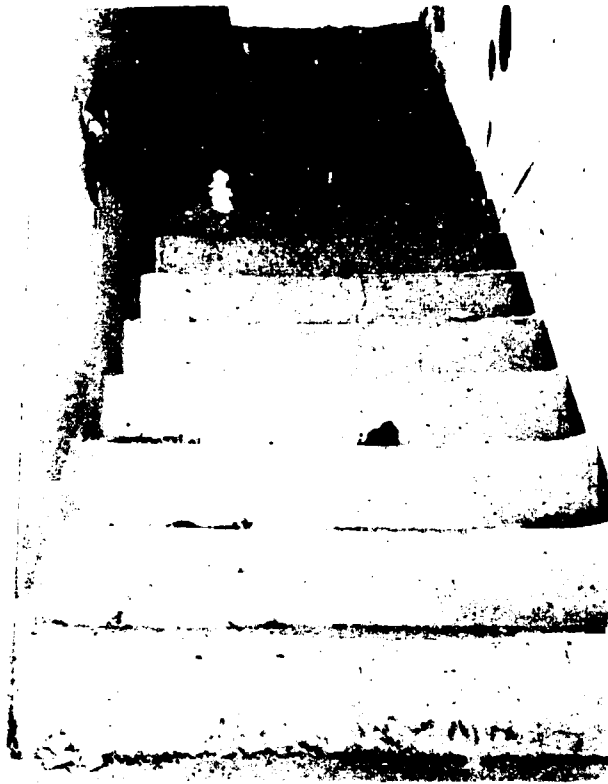
Fig. 3.71—Looking up stairs facing away from GZ (structure CAa). Note crack running up stairs and separation of construction joint.
