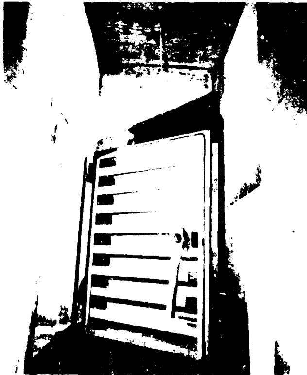
Fig. 1.26—Emergency-exit blast door (structure RC).
