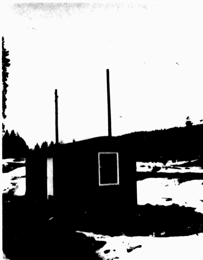
Figure 3.24 DRC hut at Falldalen
