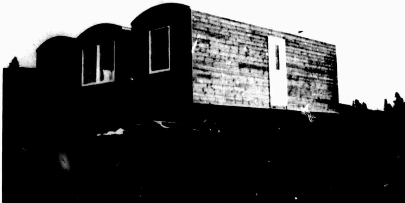
Figure 3.18 Erection of three-section Moelven house at Oyer (Refer to Figure 2.14)
