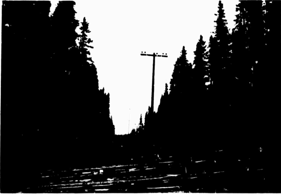
Figure 3.19 Power pole line in dense forest, wires not mounted
