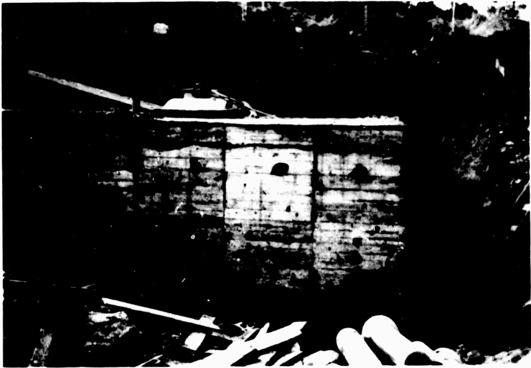
Figure 3.13 LPV before back-filling and erection of superstructure
