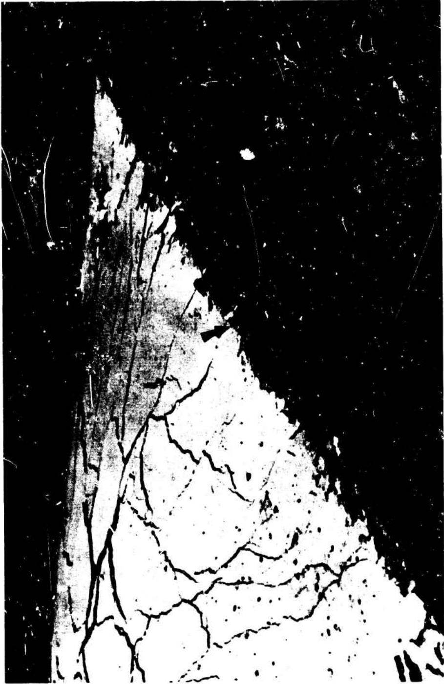
Figure E-6. Displacement of slab 4.75S1 near support at large center deflections
