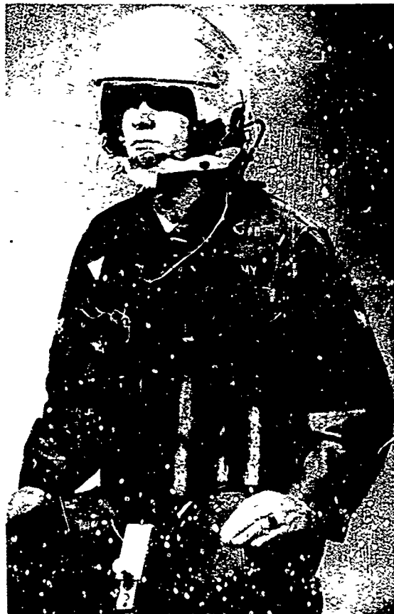
Pilot's Torso Shield with Shield Cover, Shoulder Straps and Support- ing Extension at Groin Area.
