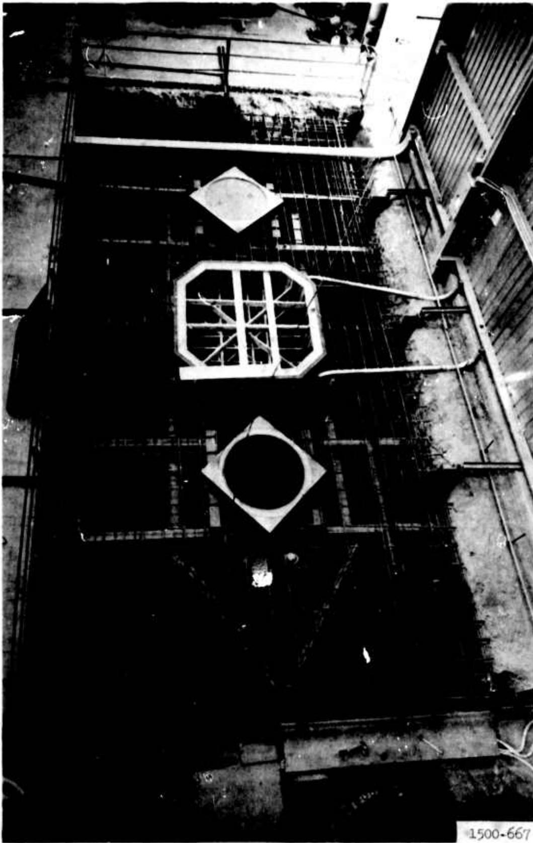
Figure 4 Construction view, 18-foot-thick foundation for SBLG.
