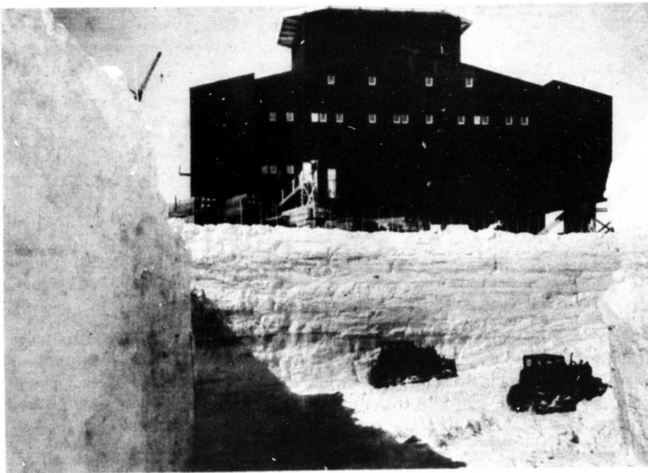
Figure 21. Bulldozers excavating a large pit at DYE-2, Greenland. The snow at this site contains heavy ice lenses. (Photo by J. McAnerney.)
