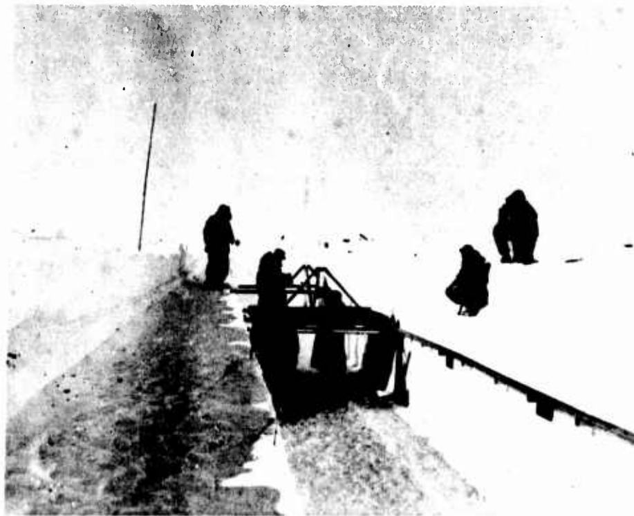
Figure 44. Arch abutments for a cut-and-cover snow tunnel. The abutments have been prepared and supports for the arch forms have been fitted. The formwork supports are acting as rails for a target trolley to guide the plow during subsequent cutting. (Photo by R. Waterhouse.)
