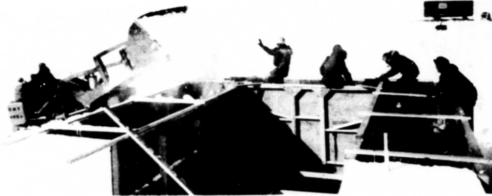
a. During construction
