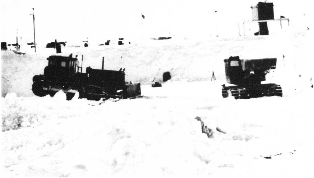
Figure 20. General excavation. Bulldozer and front-end loader excavating a building site at Byrd Station, Antarctica. (Official U.S. Navy photo.)
