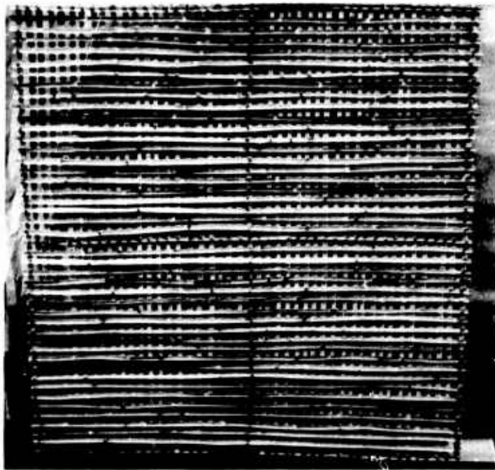
Fig. 16. Typical slab reinforcement (1-1/2 in. or 3.81 cm on center)
