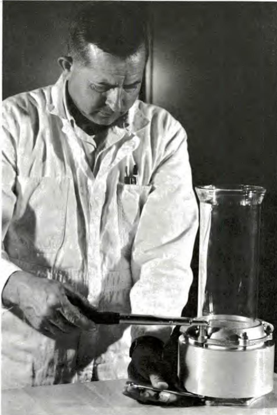
Figure 10. Use of torque wrench to avoid damage to glass pipe through uneven loading of glass flange area during assembly.
