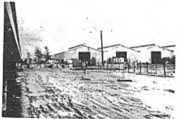
Figure 5. View of the Reefer farm at Phu Bai (Marine subsistence issue site). Refrigerated units are mobile with a temporary wooden structure built over them to keep the heat of the sun off the units. This Marine issue complex supports Navy messes in the area. Subsistence support is excellent. Most food items are plentiful and available. Ration-dense foods are used in great quantities. Foremost milk recombining plants in Danang and Chu Lai provide filled milk of excellent quality made with vegetable oil. They produced egg-nog during the holidays and are now making cottage cheese for our troops. A Marine bake shop is set up in a corner of the dry provisions warehouse to the extreme left.
