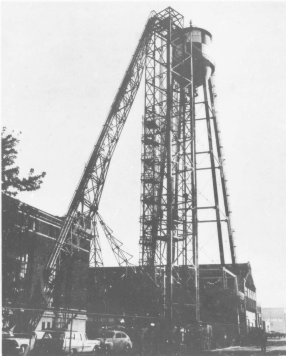
Fig. 12 Ejection Seat Facility in the foreground and Drop Tower located between it and the water tower. Aerospace Crew Equipment Laboratory, US Naval Air Engineering Center, Philadelphia, Pennsylvania, USA
