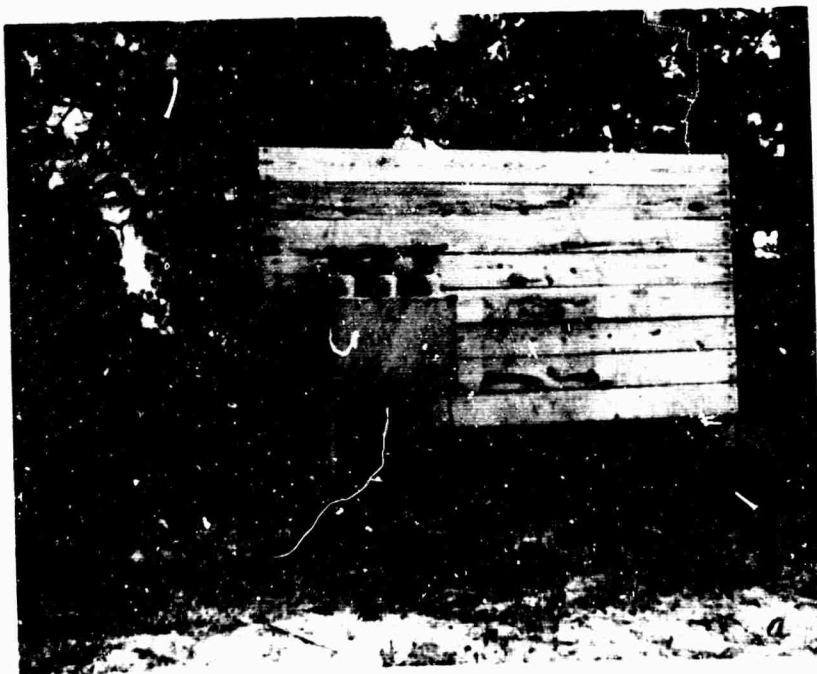
Photo No. 75 - Pre-Shot of Oil Fuse Cut-Out Panel (T-14)
