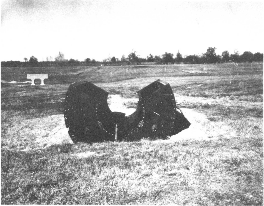
Figure 2.5 Preliminary placing operation formwork.
