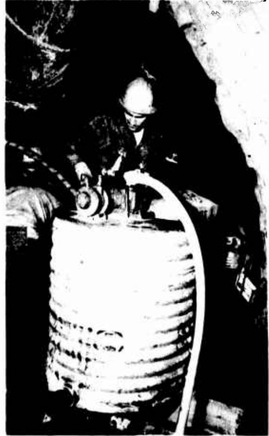
b. Tub-type grout mixer.
