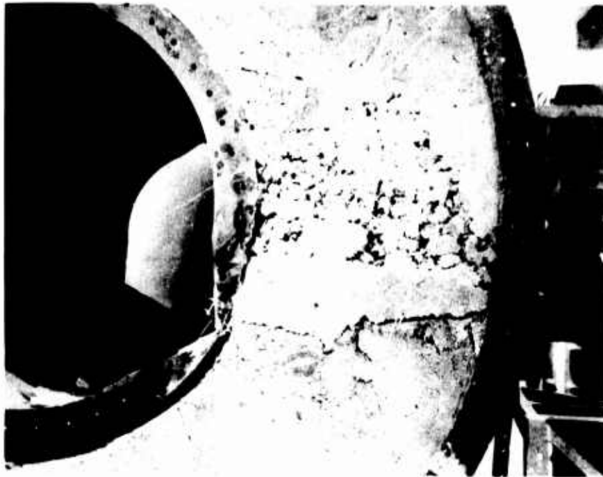
Figure 4.1 End view of vermiculite concrete section showing segregated appearance of the concrete.
