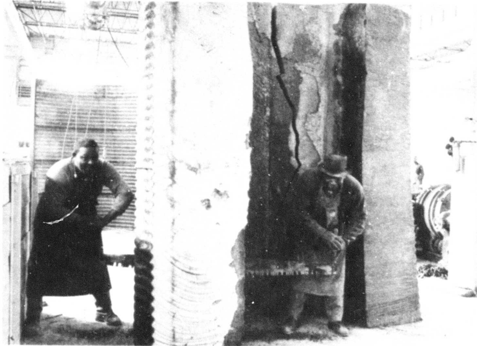
a. Handsawing of cellular concrete.
