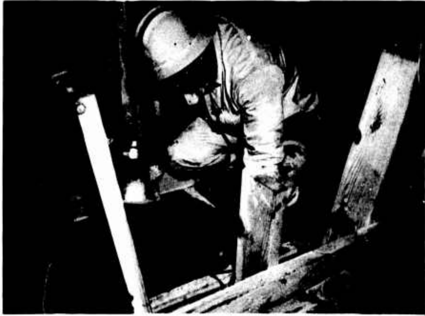
a. Overall view of opening.
