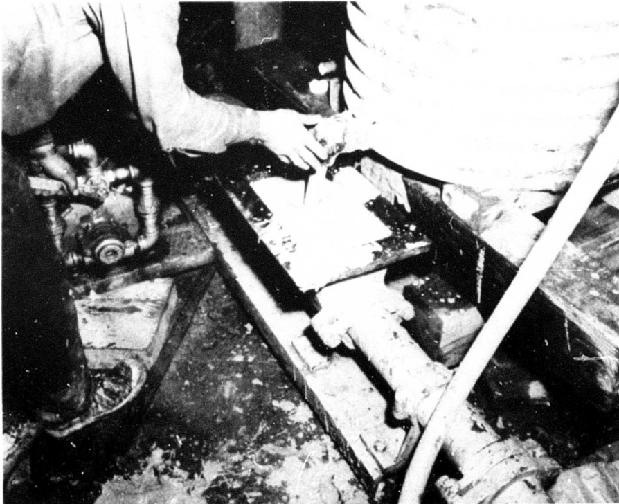
Figure A.3 Cellular concrete discharging into an open-throat pump.
