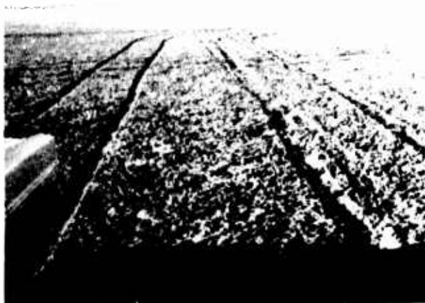
Figure 12. Comparison of Tire Ruts Made in November 1966 (Left) and October 1962 (Right) in a Soft, Dry Friable Surface. It appears that this area was not flooded in contrast to most of the barren playa, and consequently was virtually unchanged.
