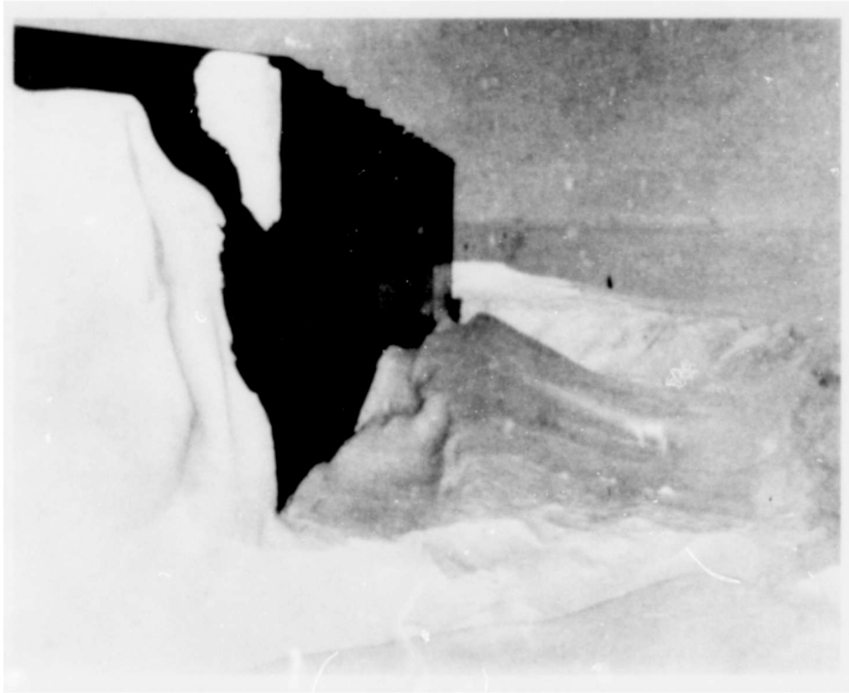
Figure 11. Drift snow around the NCEL T5M shop building after 1 year of accumulation (looking south).
