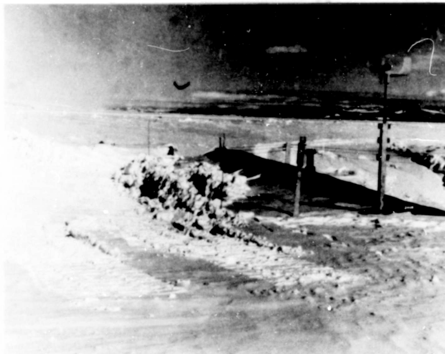
Figure 7. NCEL camp after 4 years of drift accumulation; note upwind portion of the trench to right of Jamesway (looking south).
