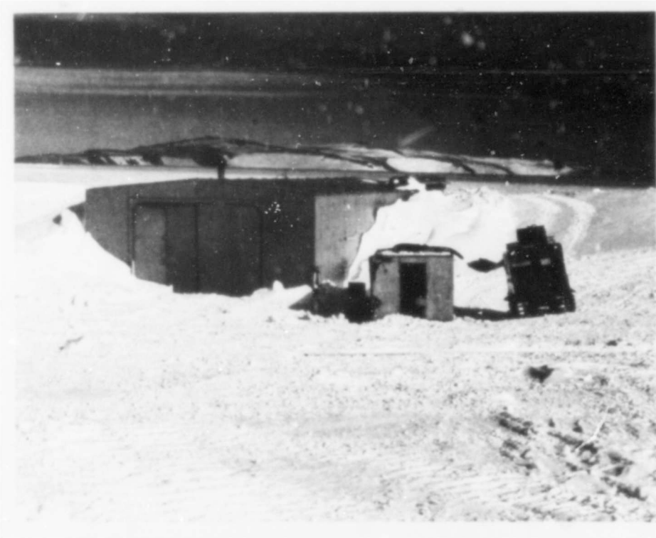
Figure 14. Drift around T5M after 4 years of accumulation; the area in front of the doors has been cleared (looking south).
