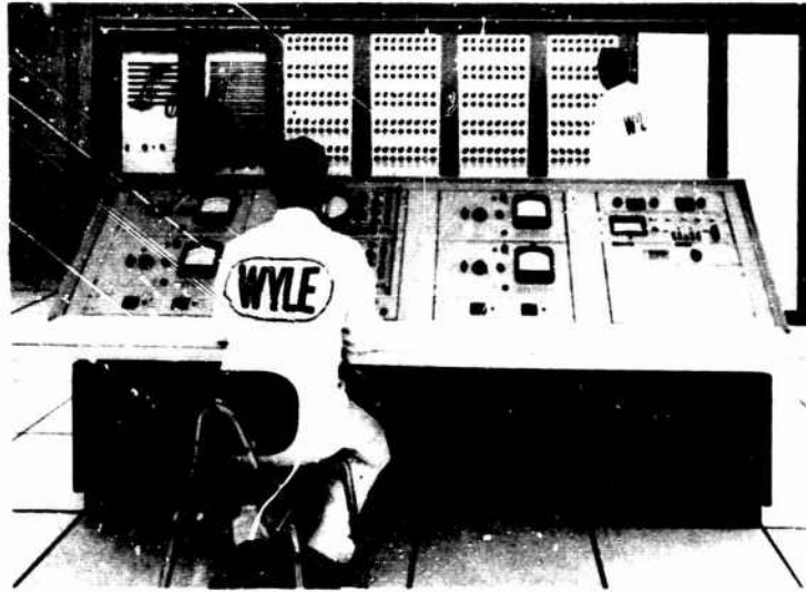
Fig. 8. Charge amplifiers in instrumentation room
