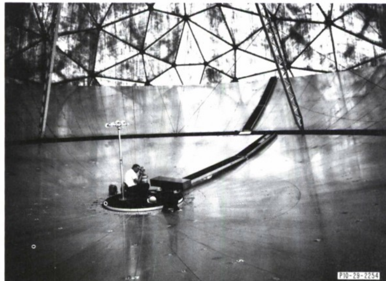
Fig. 18. Photograph showing instrument and stanchion, front access catwalks, operator's chair, platform and lights.
