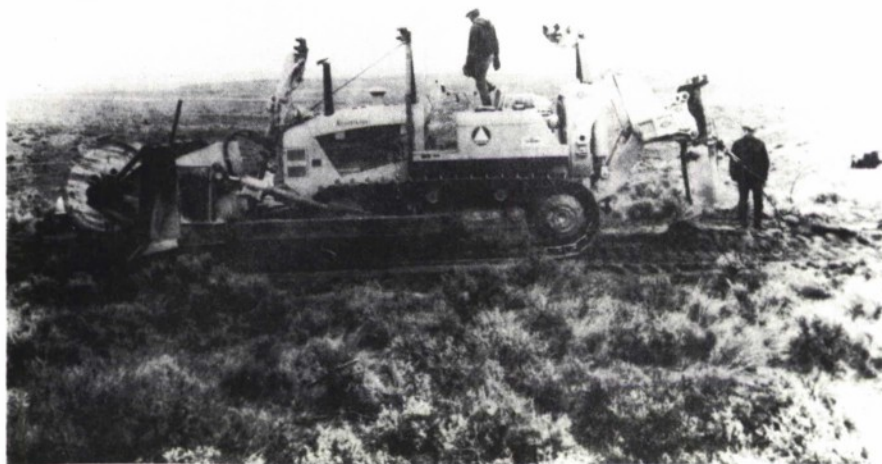
Figure 9 Trenching Rig in Use at E3
