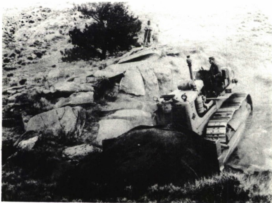
Figure 5 Cable Route Preparation at E3 Leg 1
