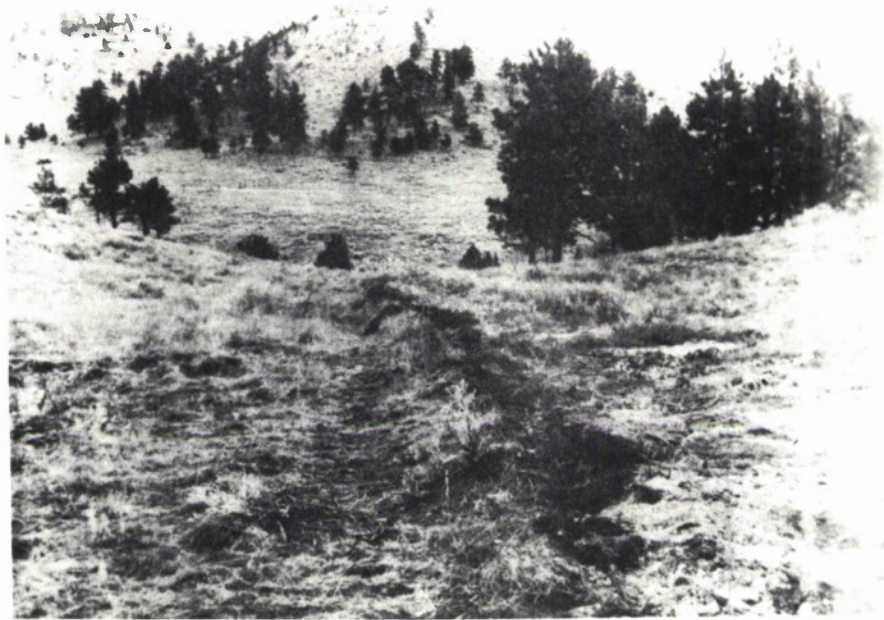
Figure 8 Completed Cable Trench at E3
