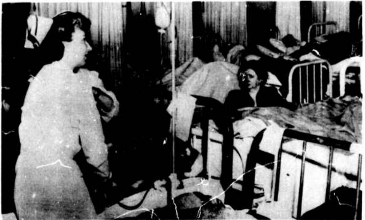
Above: A nurse in Perth Amboy General Hospital administers aid to one of the victims of the explosion. In other beds are additional casualties of the blast.
