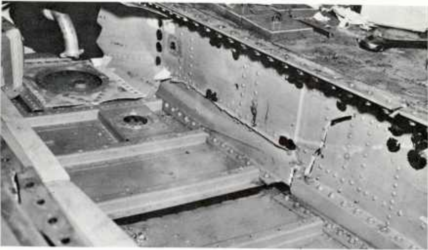
FIGURE 10.—Fatigue failure of wing main spar—growth through areas of stress concentration (see also fig. 11).
