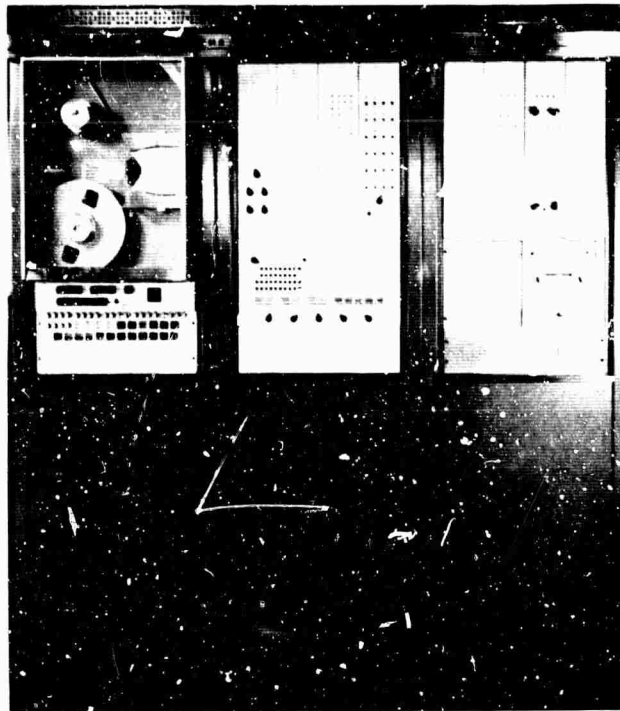
Fig. 1 - Digital data recording system installed at the Randle Cliff Radar facility at the Chesapeake Bay Division of NRL. The left cabinet contains the magnetic tape recorder/reproducer and a radar range digitizer (not described in this report). The center cabinet contains the linearizer, digital multiplexer, sequencer, and analog/digital converter plus the main system display and control panel. The right cabinet contains the analog multiplexer, the data search and selected readout, and the format generator.
