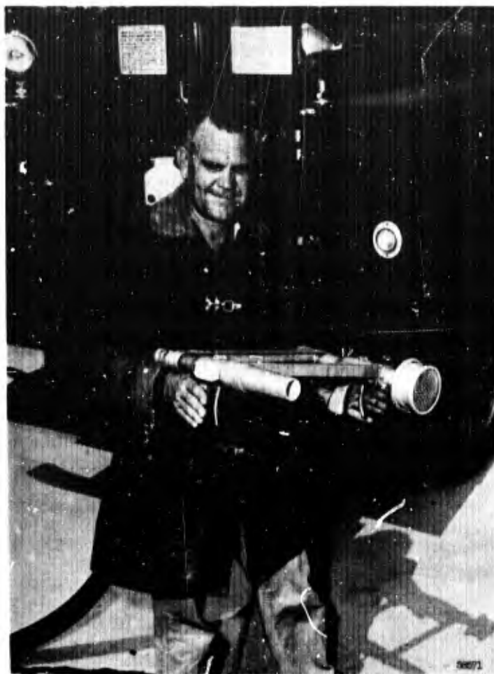
Fig. 2 - A close-up of the dual nozzle with finger-tip control valves. Light Water is on the operators left side.
