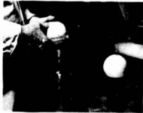
a. b. Figure 7. The riser explosive is removed and the top of the charge is scraped smooth.
