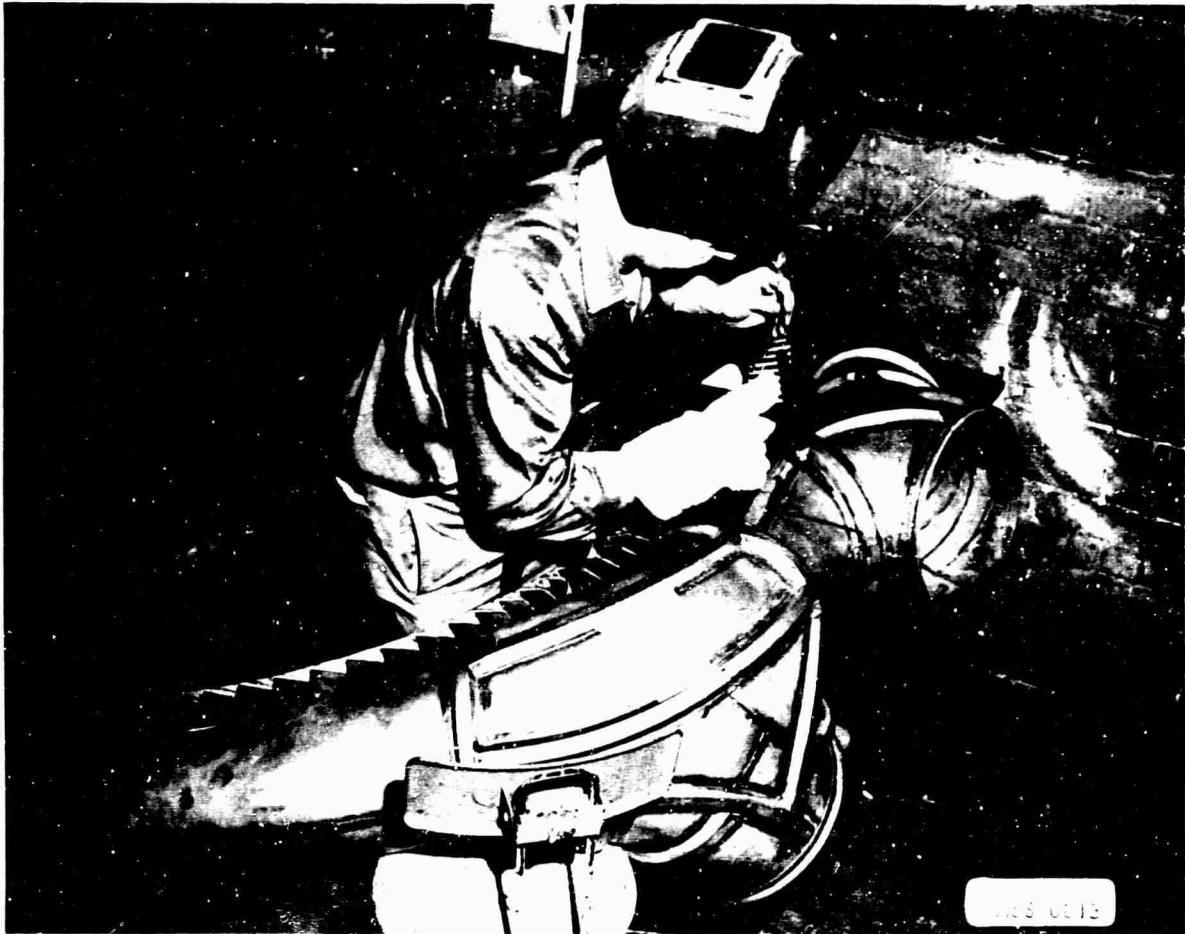
Figure I-80. Hat Section Added To The Lift Fan Scroll
