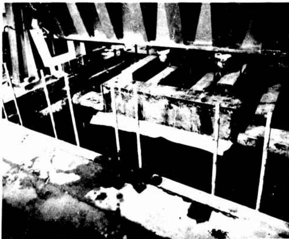
Figure 3. Inflatable bag wrapped in canvas with Teflon rub-sheet in place between footing and bag.
