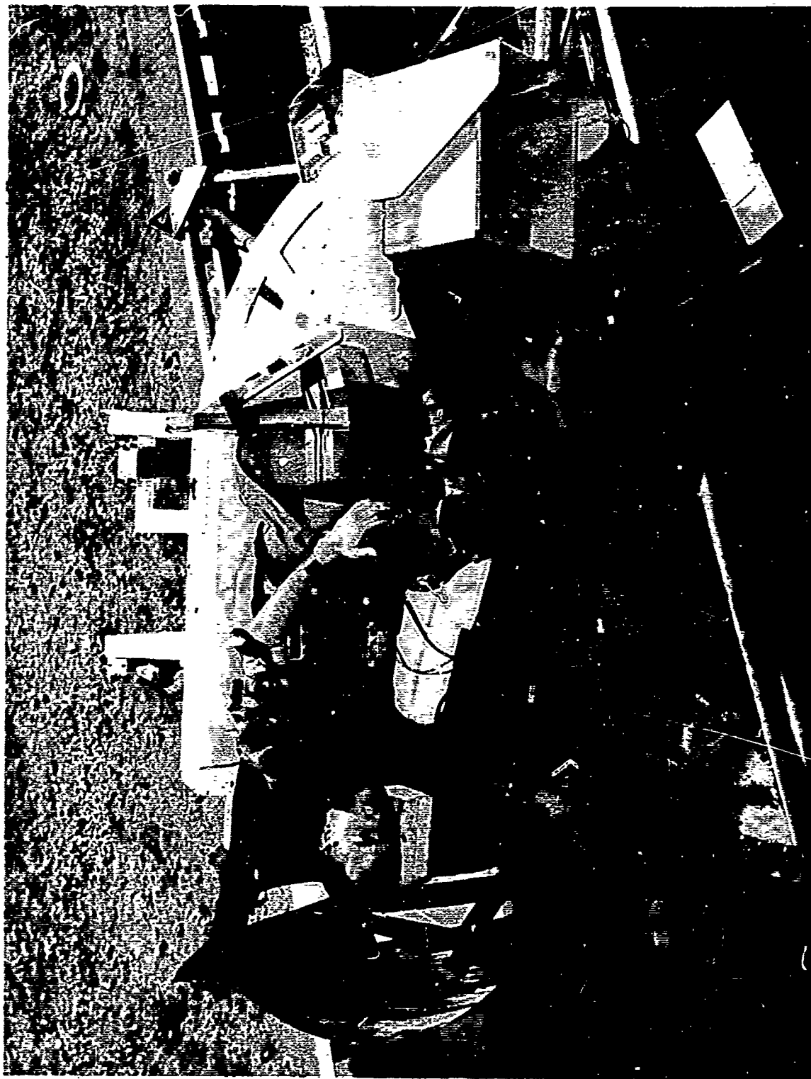
Figure 3. Sled Number 1 with Volunteer Test Subject. Direction of motion is from left to right. Note that the subject was required to lie on his side when this sled was used.
