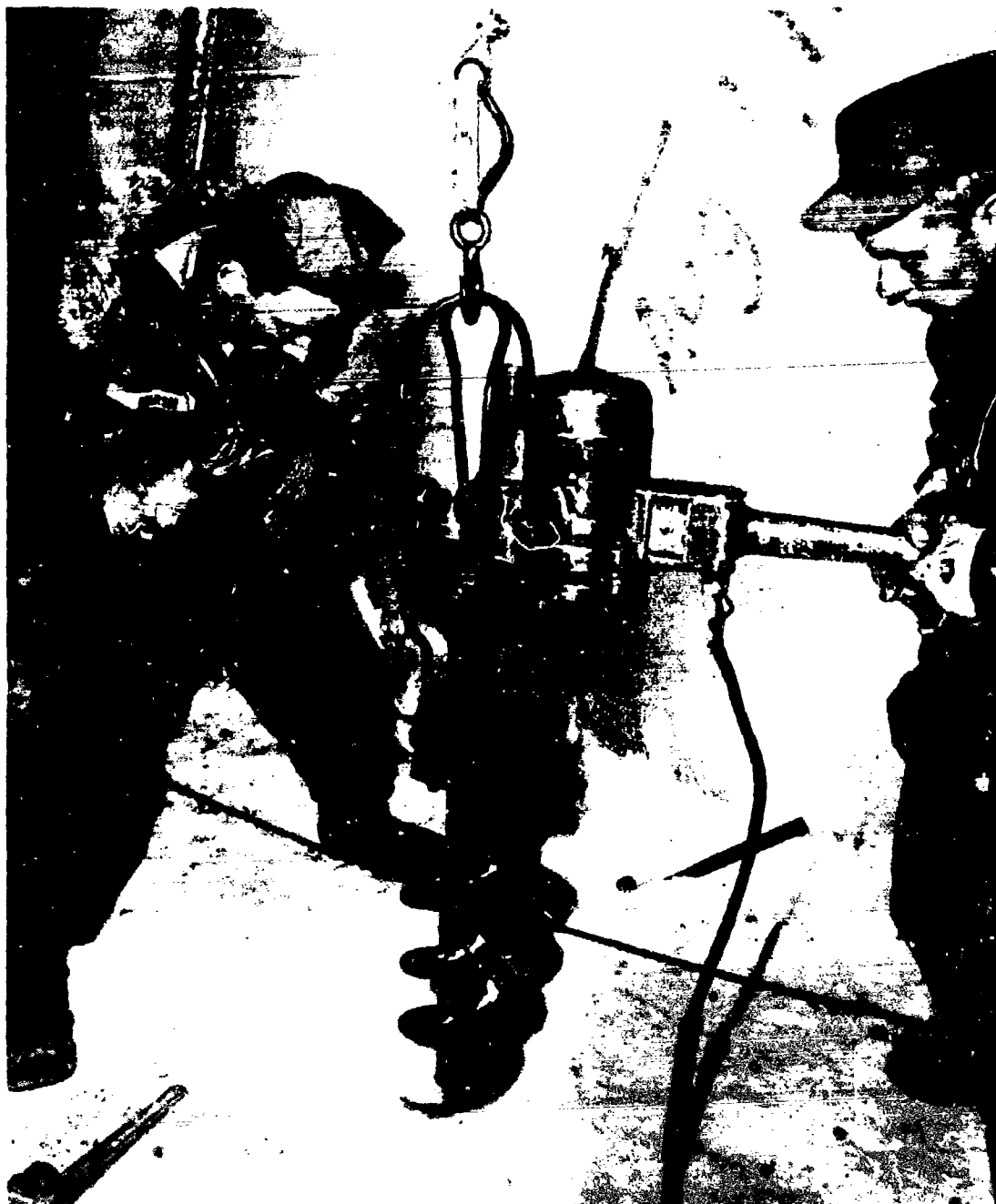
Figure 6. Augering hole in ice floor preliminary to installation of 4 x 4 underpinning post.
