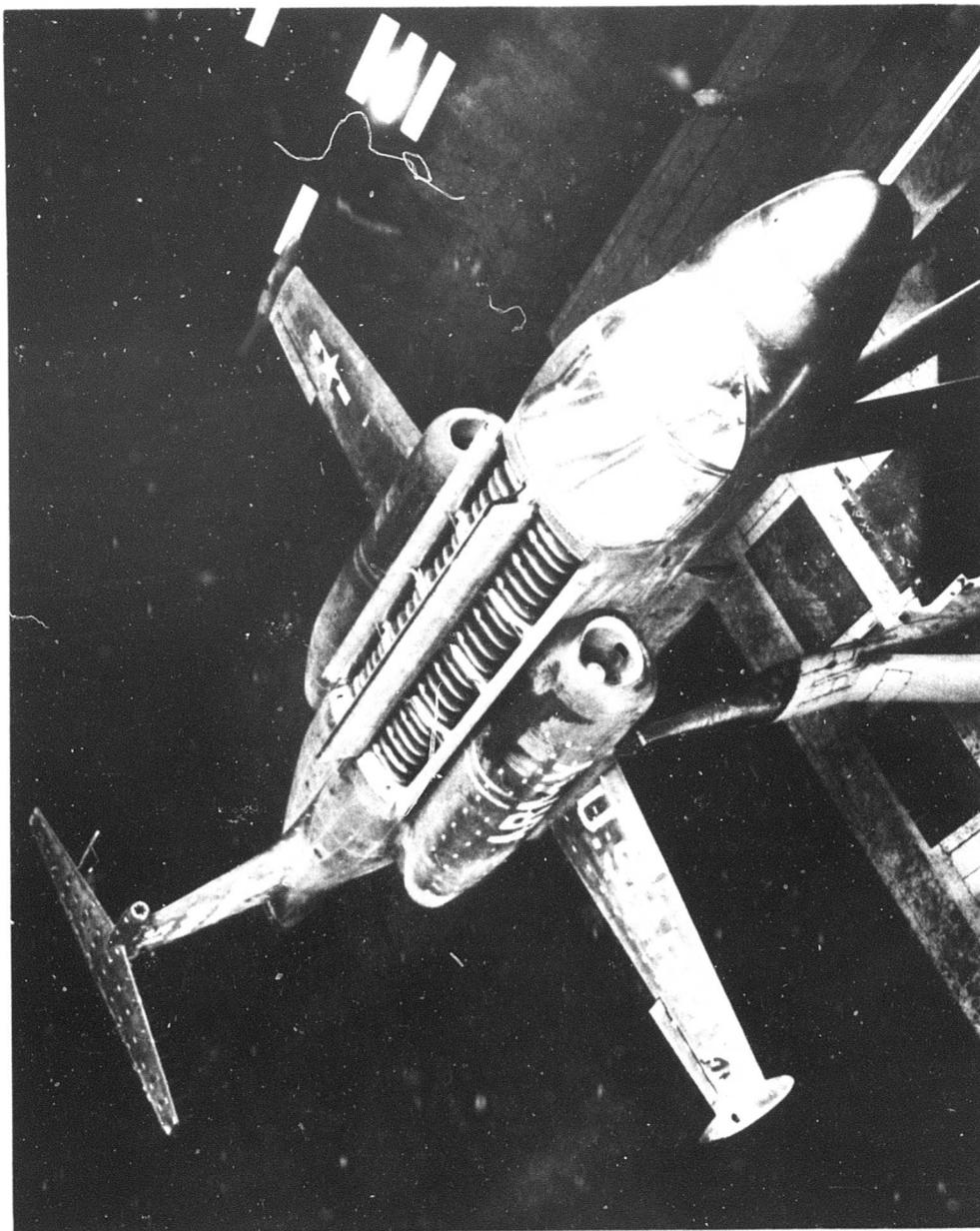
Fig. 4 The Lockheed XV-4A mounted in the Ames 40 ft by 80 ft wind-tunnel
