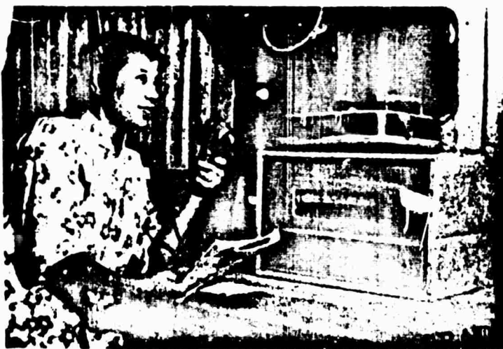
A communal wired station in the mountainous region in Fukien. This is the second type of wired broadcasting we described above. (The picture is adopted from Wuhsientien (Radio) , No. 1, 1960).
