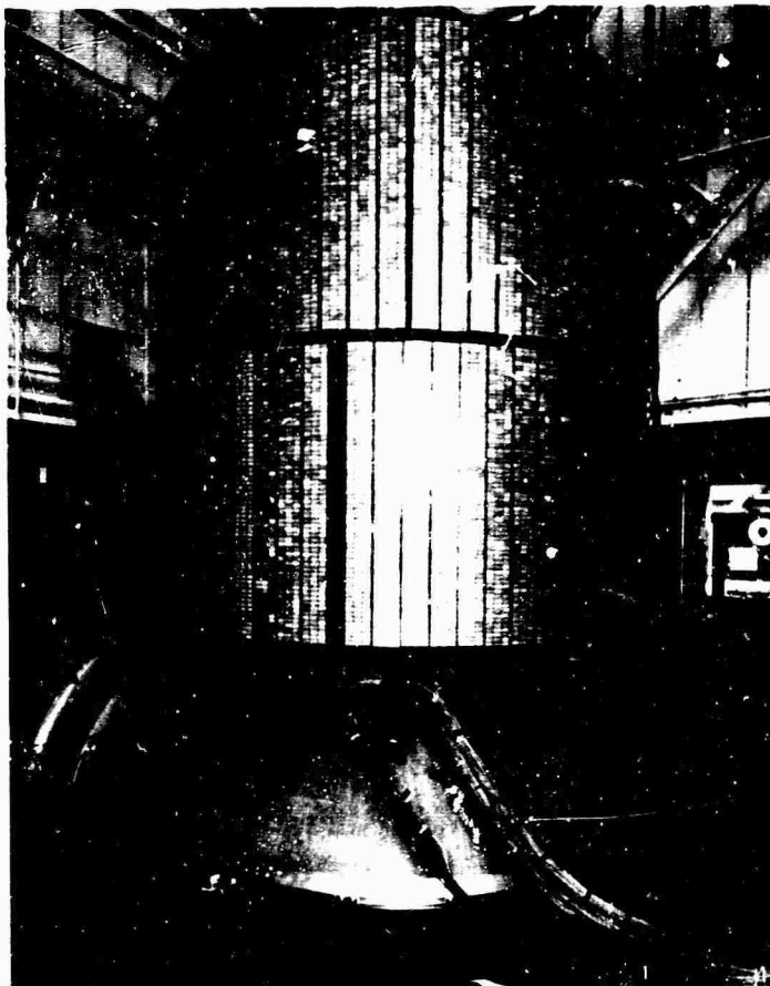
Fig. 16 - Spacecraft-adaptor configuration during lateral qualification testing
